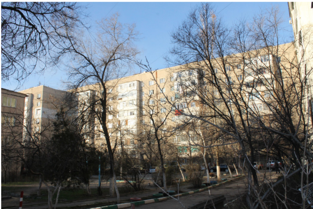
Figure 9.3: View of the back of building 37.
