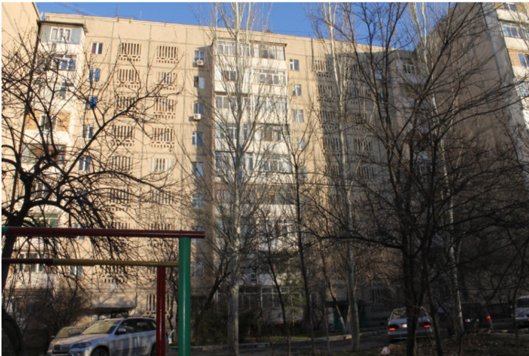
Figure 9.5: Front view of building 43.
