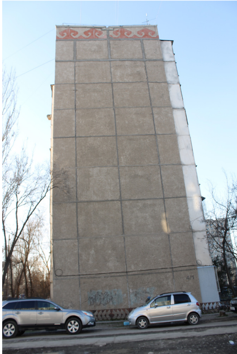
Figure 9.13: Lateral view of building 4/1.
