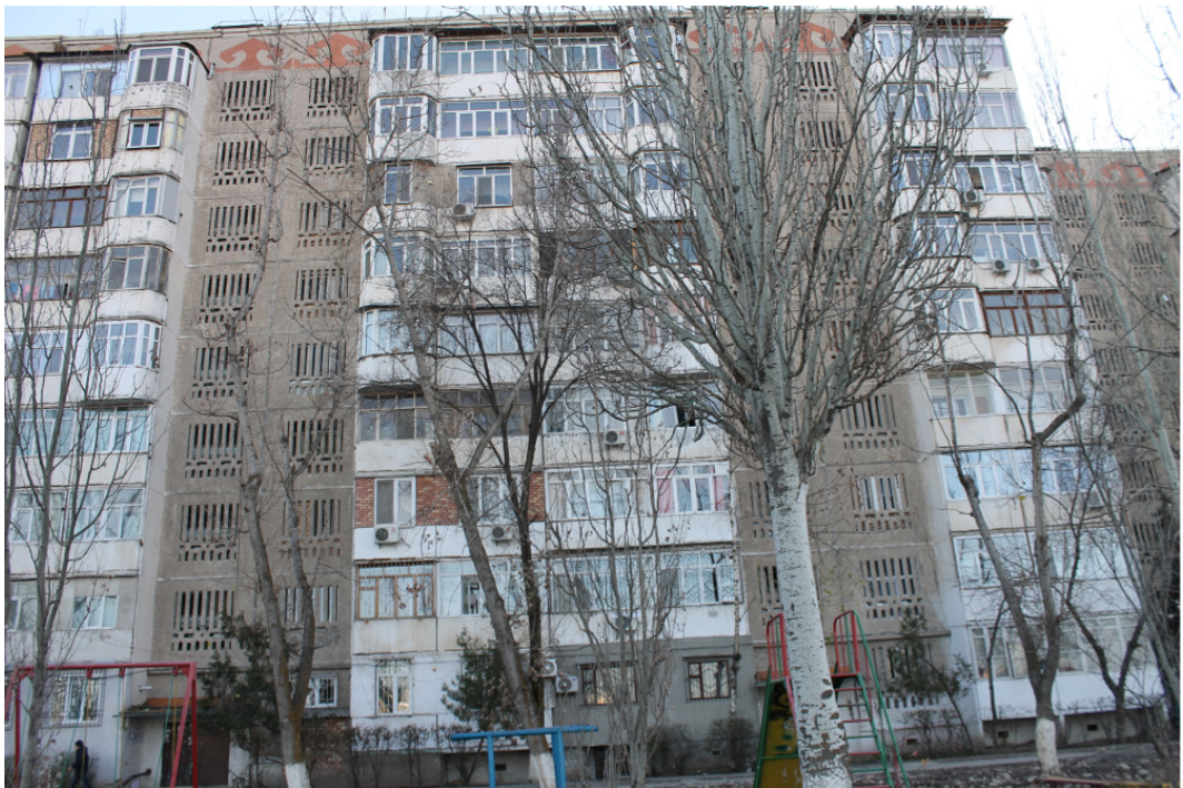
Figure 9.1: Front view of building 37.
