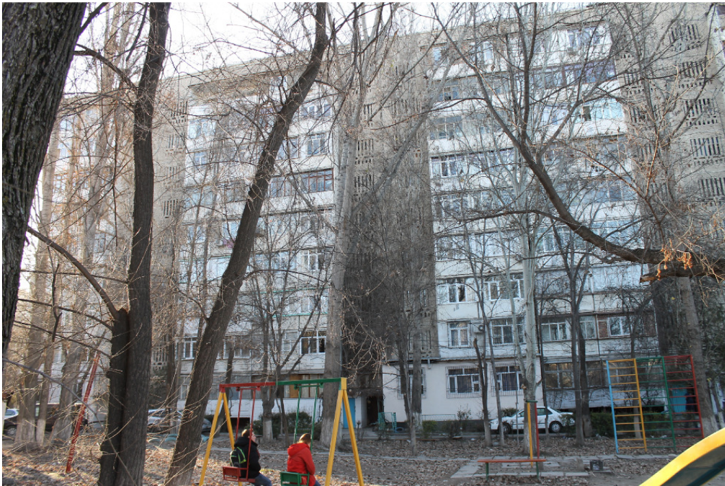
Figure 9.10: View of the back of building 25.
