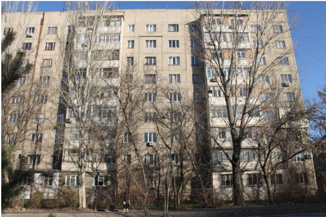
Figure 9.8: Front view of building 25.
