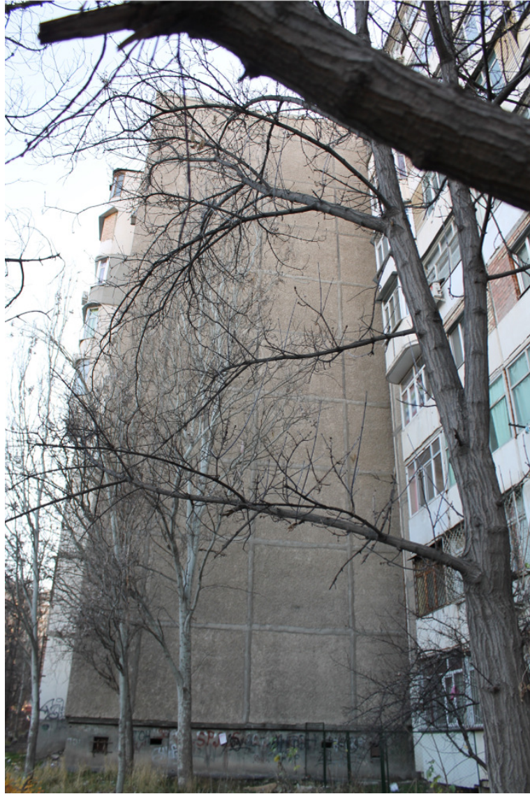
Figure 9.6: Lateral view of building 43.
