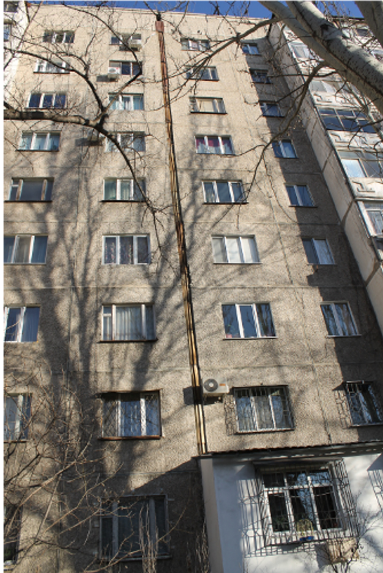
Figure 9.11: View of the seismic joint in building 25.
