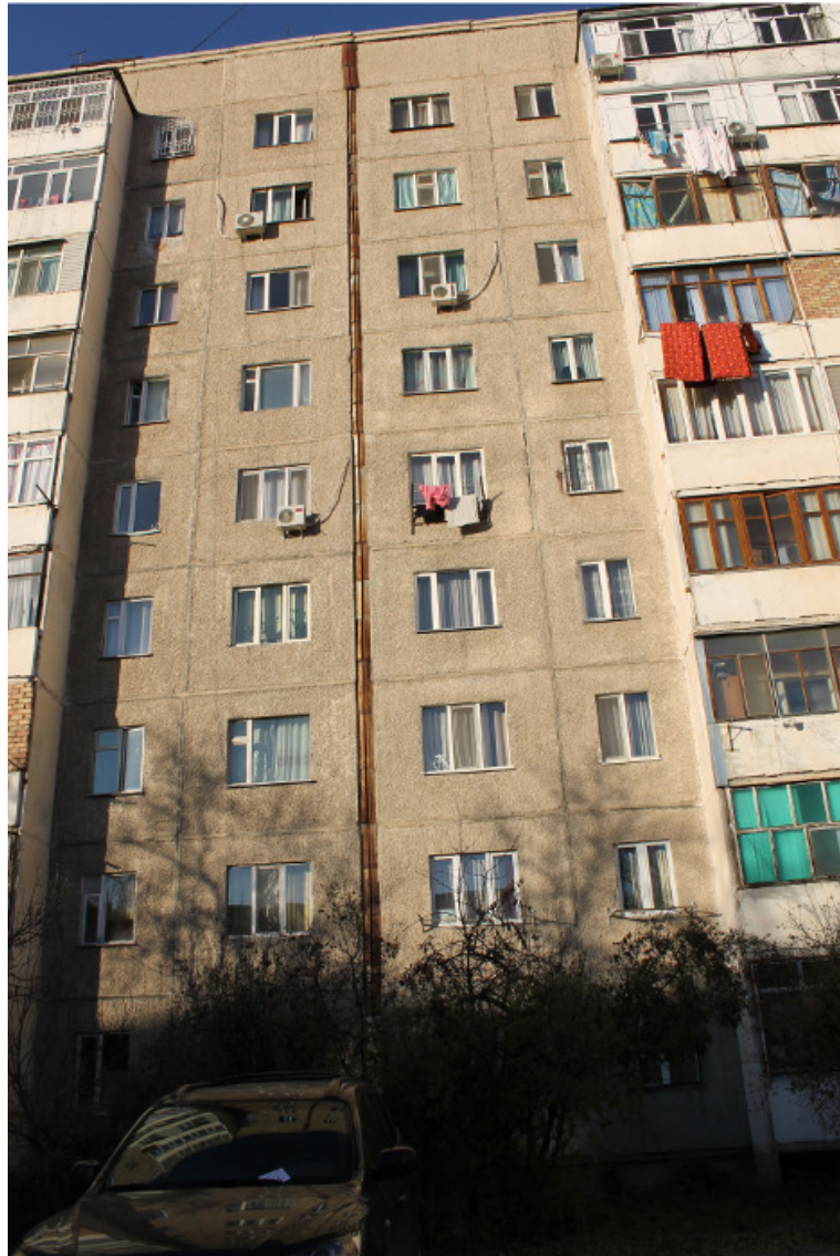
Figure 9.4: View of the seismic joint in building 37.
