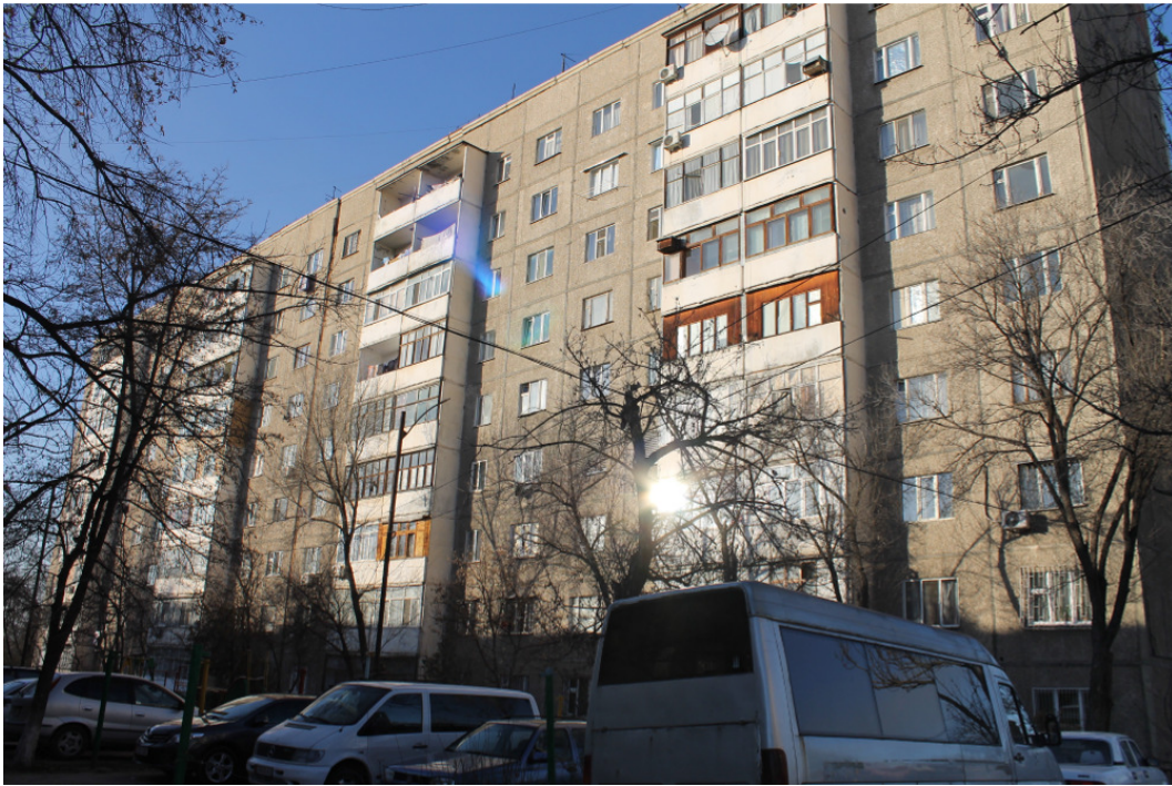
Figure 9.14: View of the back of building 4/1.
