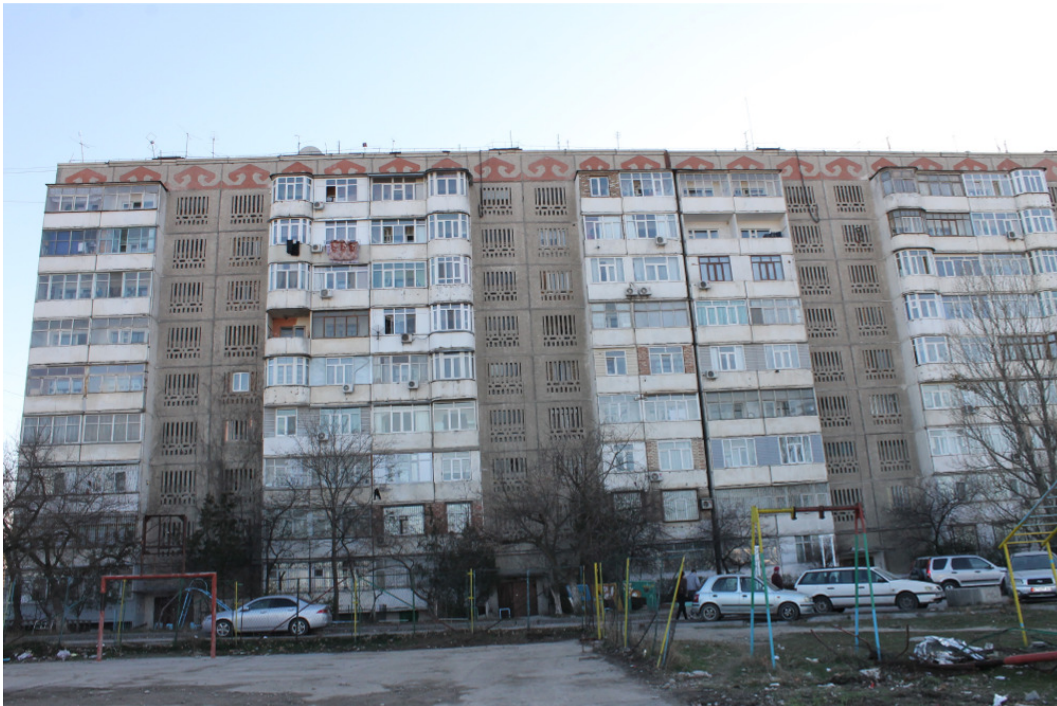
Figure 9.12: Front view of building 4/1.
