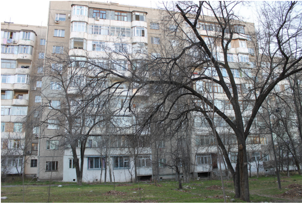
Figure 9.7: View of the back of building 43.
