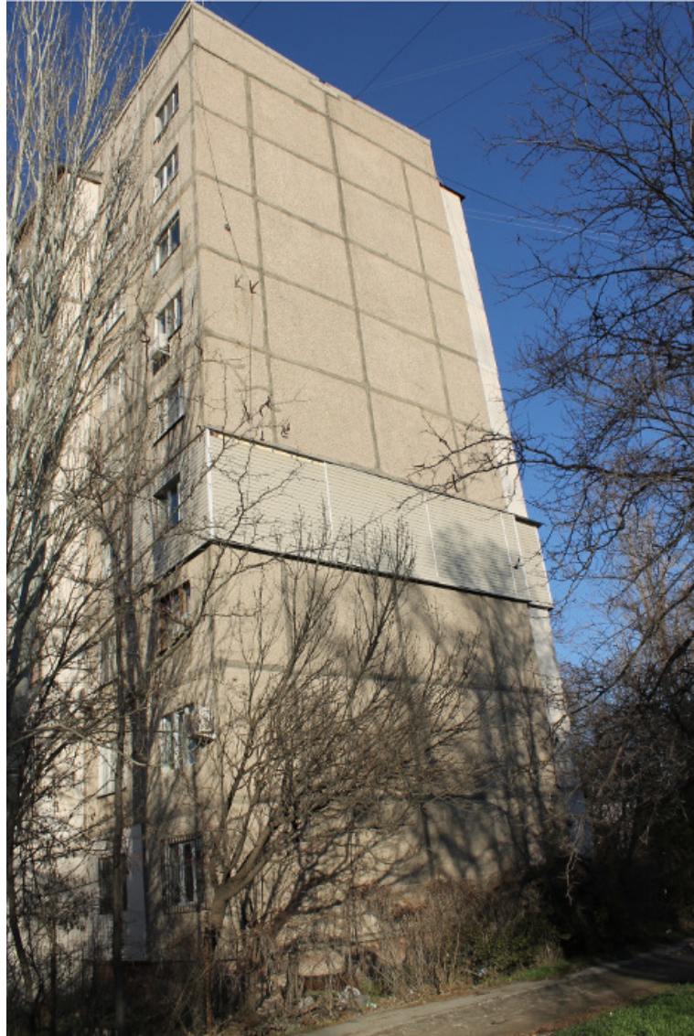
Figure 9.9: Lateral view of building 25.
