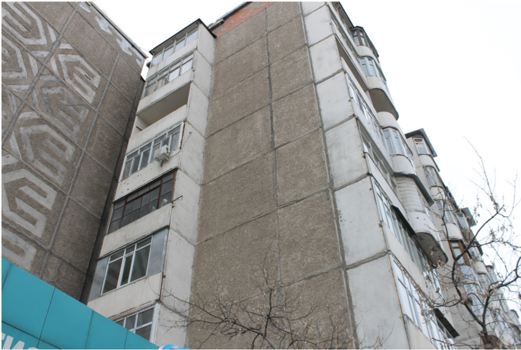
Figure 9.2: Lateral view of building 37.
