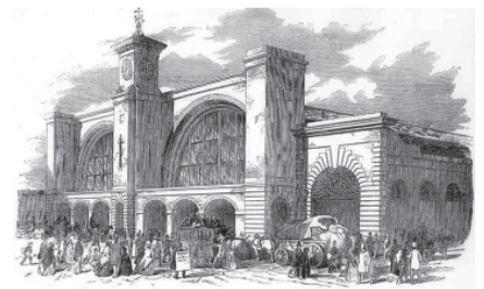
Fig.6 Lewis Cubitt, King's Cross station , Londra, 1851- 52
