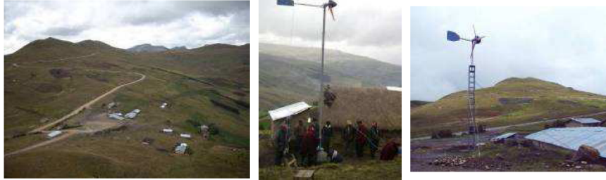
Figure 2.6: Installation of 100 W and 500 W wind generators in El Alumbre
