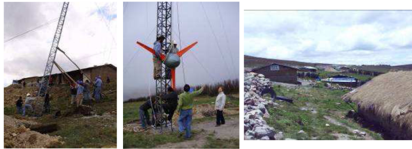
Figure 2.4: Installation of 500 W wind generator in Alto Peru
