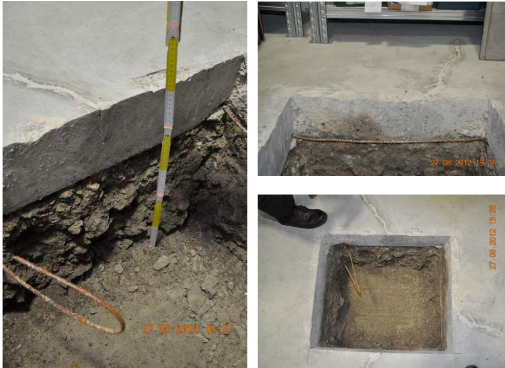
Figure 4.42 N° R.G. 10141 Example of in-situ survey
