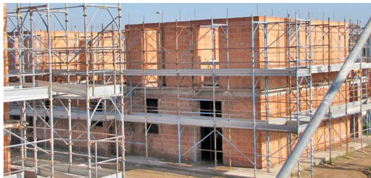
Figure 6.52 Example of masonry structure
