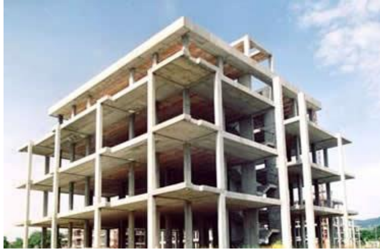
Figure 6.49 Example Reinforced concrete structure
