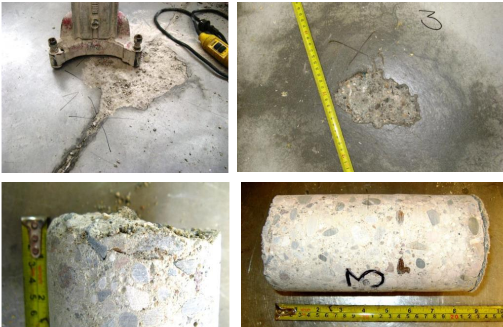
Figure 4.38 N° R.G. 6314 sampling of the inner concrete flooring
