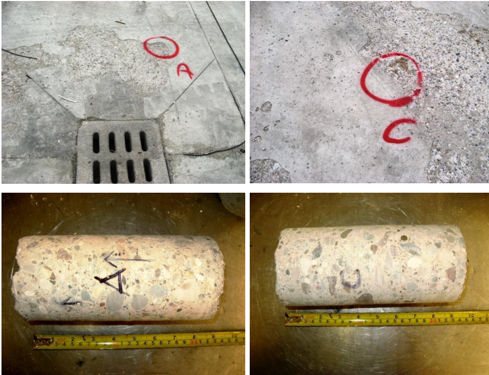
Figure 4.39 N° R.G. 6314 sampling of the outer concrete flooring
