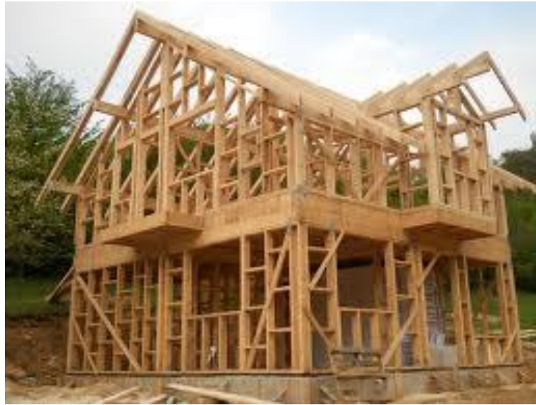
Figure 6.51 Example of timber structure
