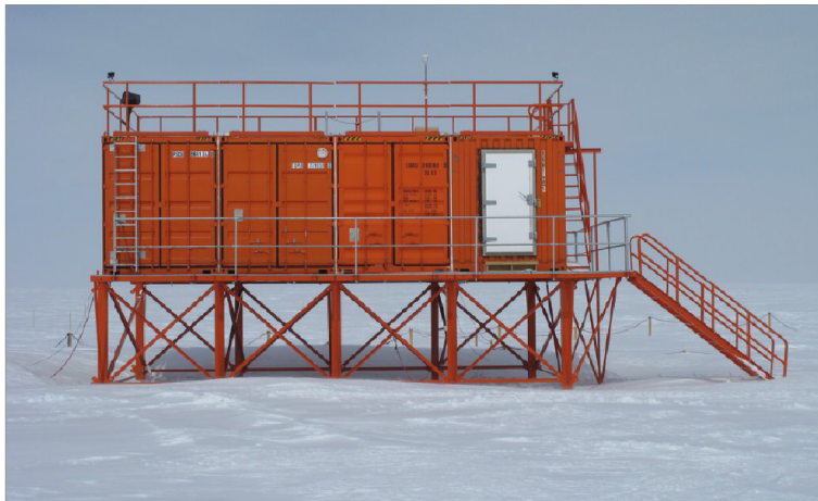
Figure 3.0.2: Physical Shelter where Lidar system and REFIR-PAD instrument are located and on which the VAISALA station is set
