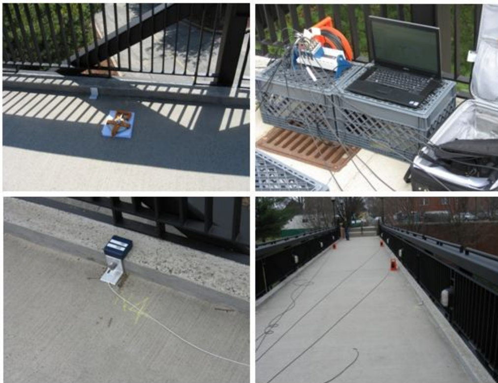
Figure 1.6 April test data acquisition system and bridge instrumentation
