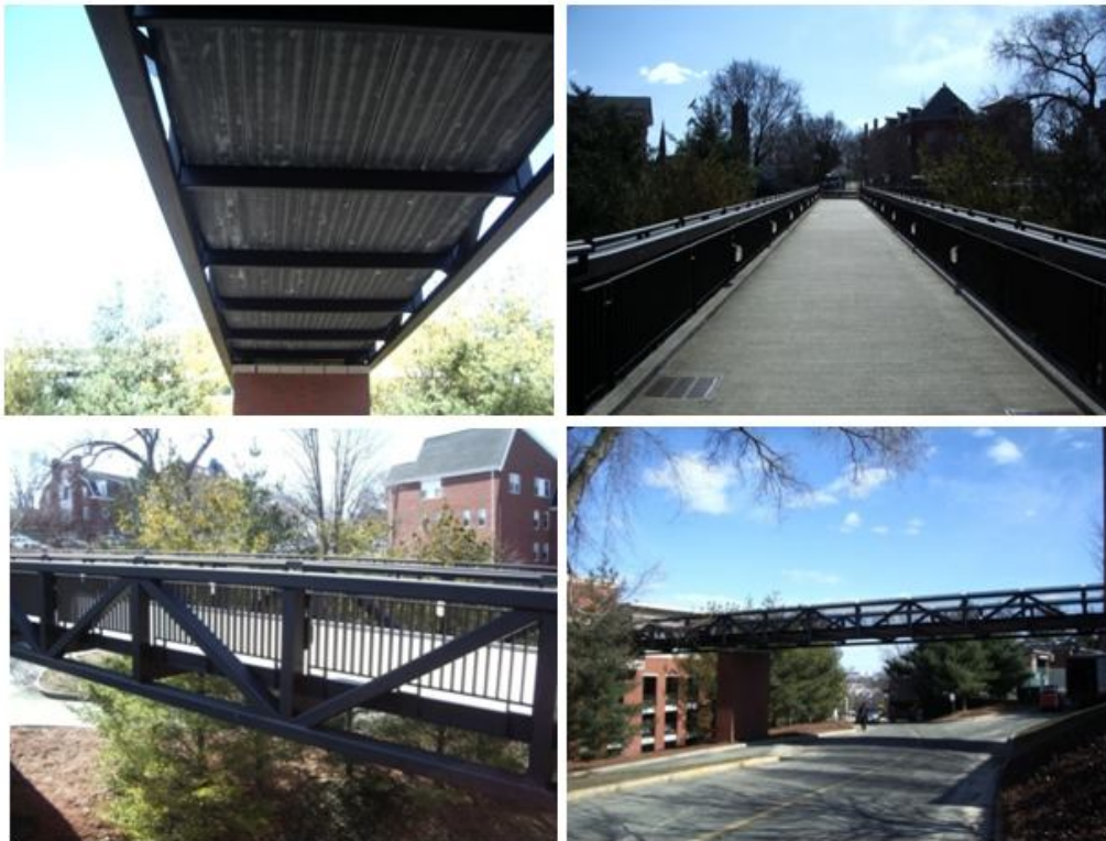
Figure 1.1 The Dowling Hall footbridge
