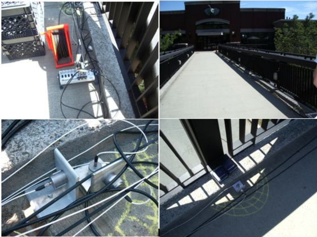
Figure 1.8 June test data acquisition system and bridge instrumentation
