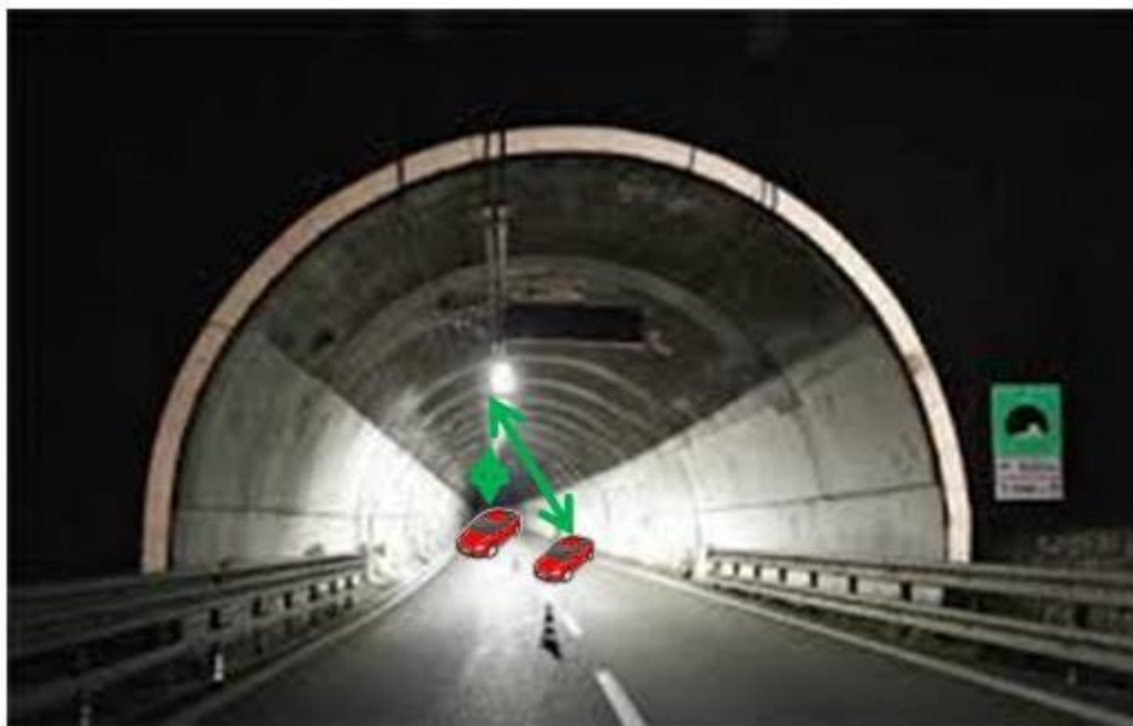
Figure 50: VLC as AP in a tunnel.
