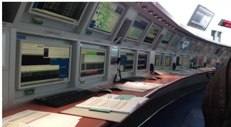
Figure 5: MSG Control Room
