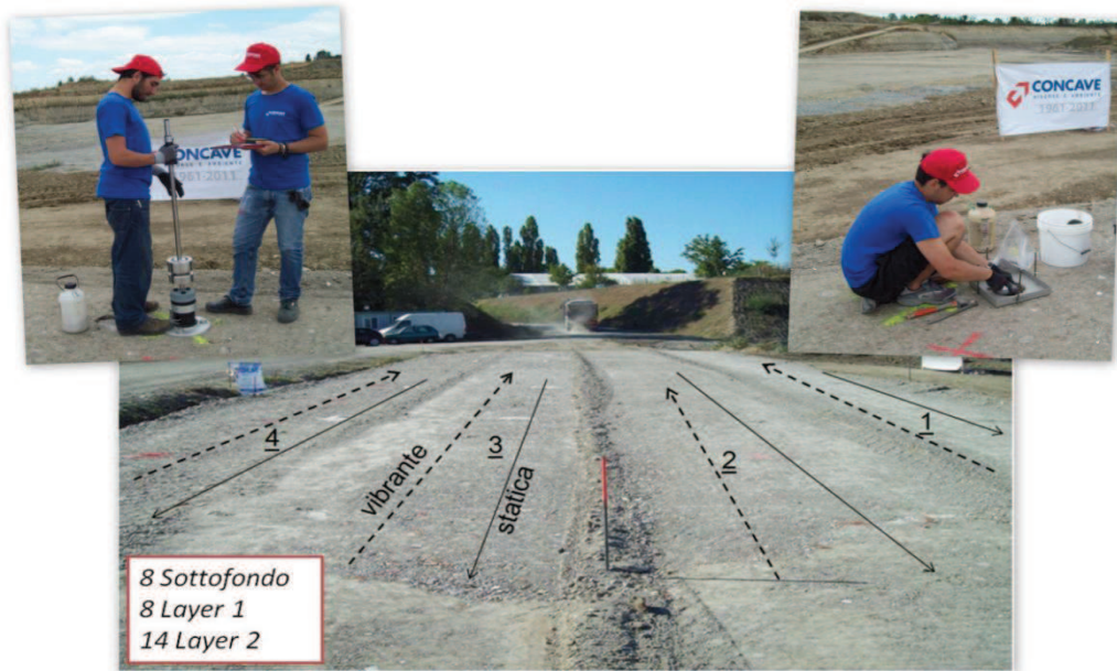
Figure 5.11. roller passes and test phases for each lift.
