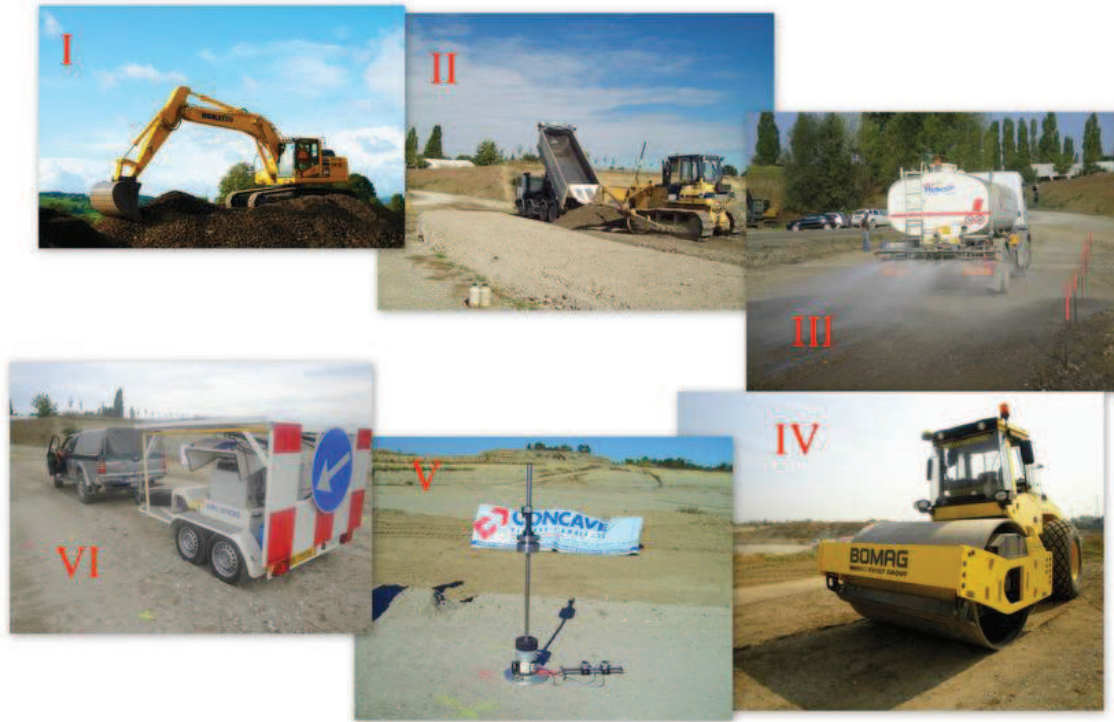
Figure 5.10. Construction and testing devices.
