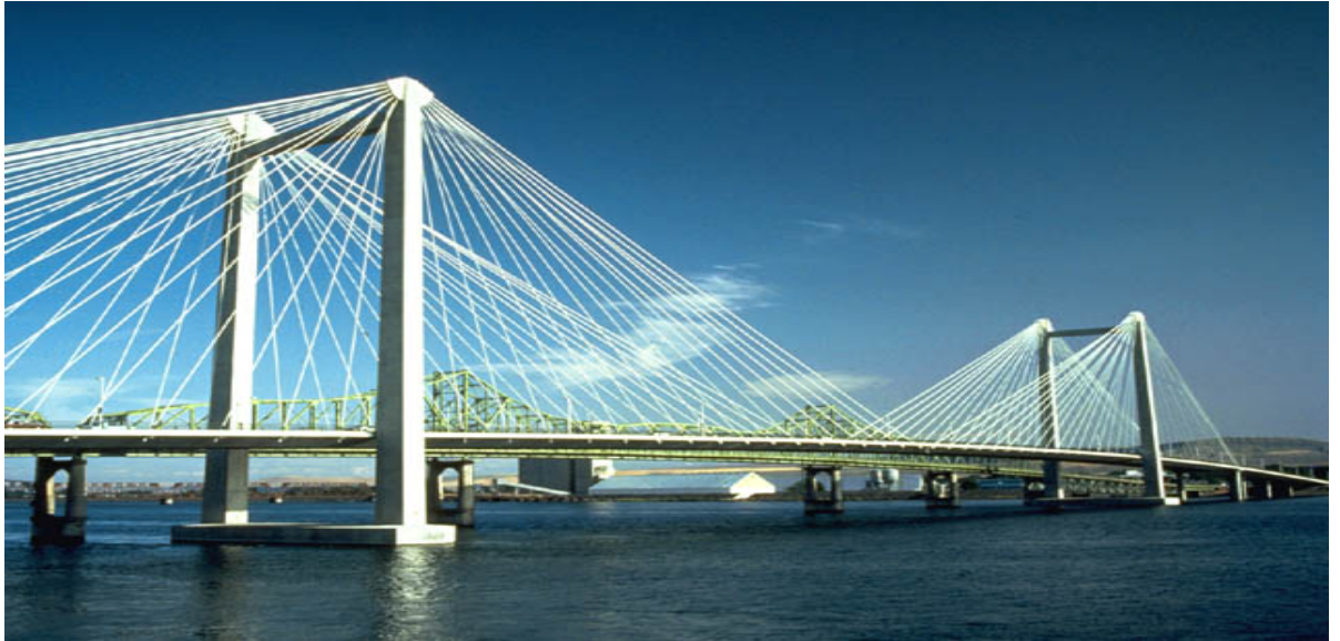
Figure 1.3. A view of the Pasco-Kennewick Bridge
