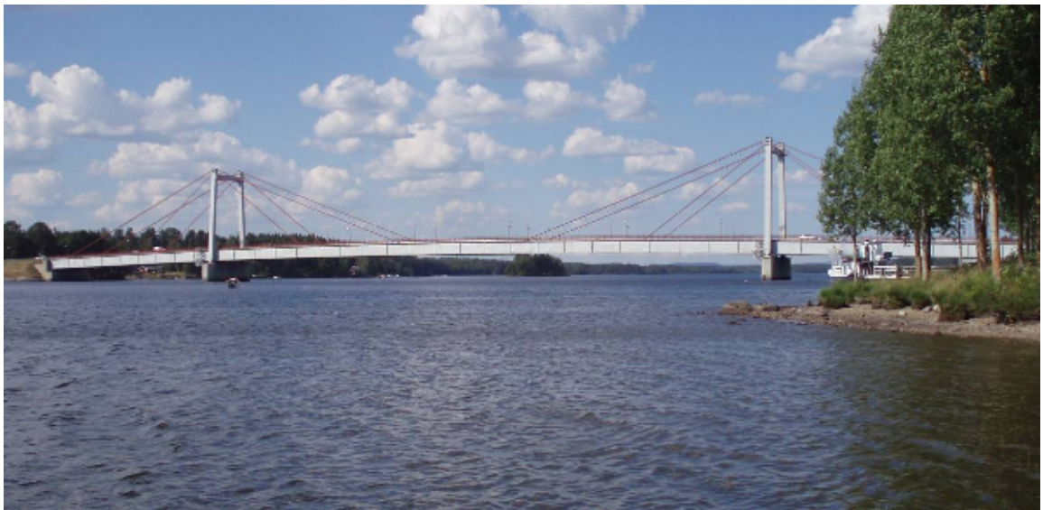
Figure 1.2. A view of Stromsund Bridge in Sweden
