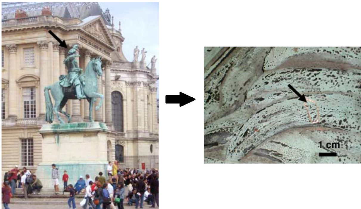
Figure 14: green streaking and discoloration phenomenon on the statue of Louis XIV. The picture on the right shows the presence of blackish areas and island [28]
