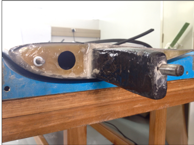
Figure 8.6 – Damage at the bonding line of the root rib and at the front spar web out of the wing after Test 3.
