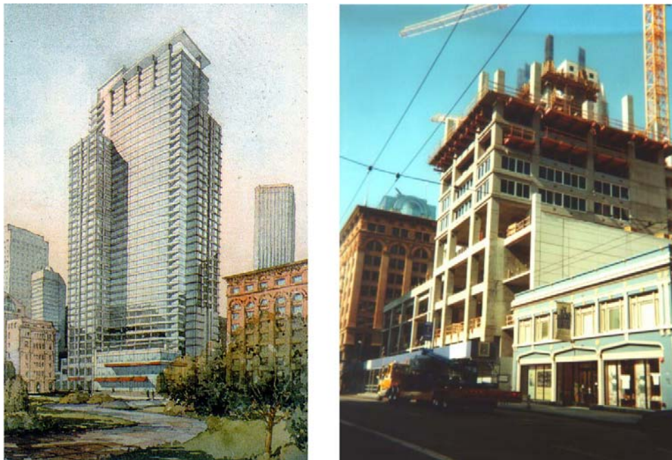
1.15 Figure – From theory to practice. 39-storey apartment building in San Francisco, Paramount Building, equipped with rocking frame connection [35, 37]
