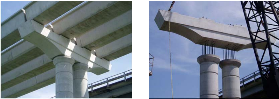
1.16 Figure – Lake Belton Bridge, Texas-U.S.A.
