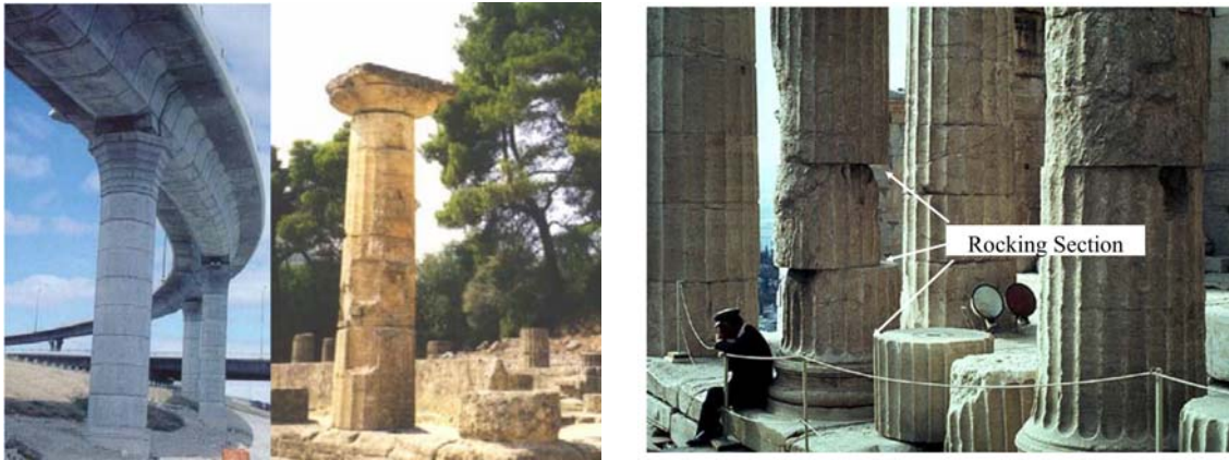
2.1 Figure – The real origin of rocking systems self centering and limited damage response under earthquake loading [57]
