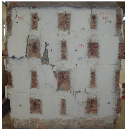
Figure 7.19 Cracking pattern of one compression test CC14_01
