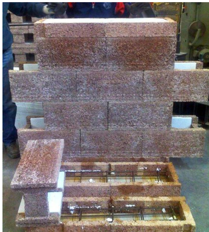
Fig.2.4 Disposition of the blocks for the creation of the grid-wall of the Lab.Tests
