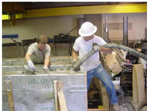
Figure 1.4 – Concrete casting phase
