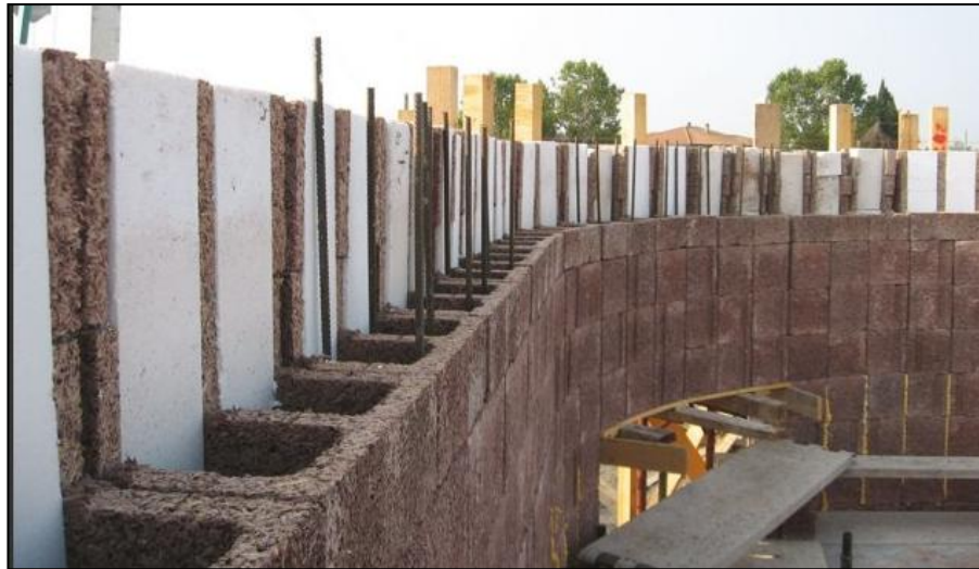
Figure 1.3 – Shear Type grid walls during construction phase
