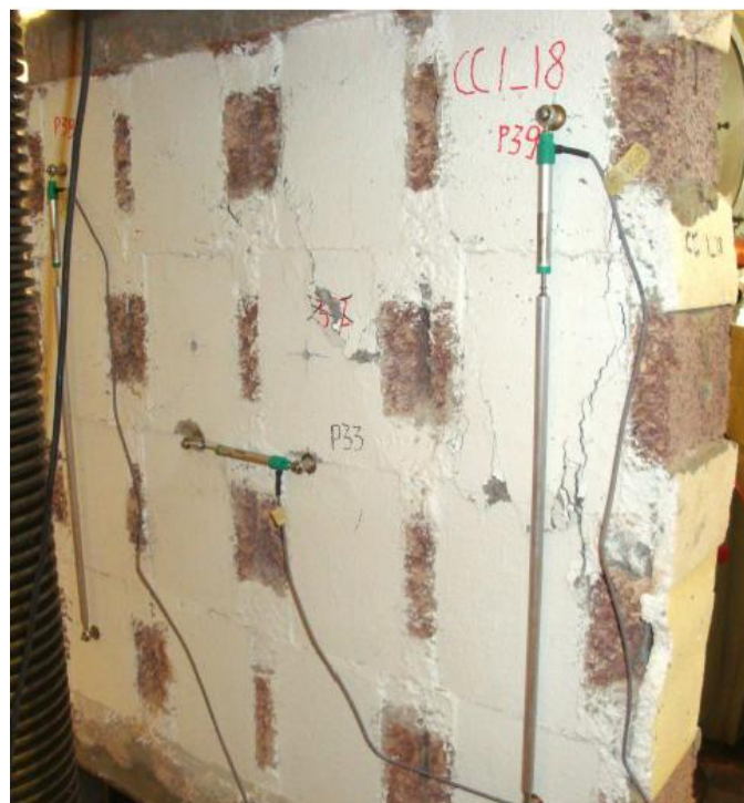
Figure 7.22 Cracking pattern of one compression test CC1_18
