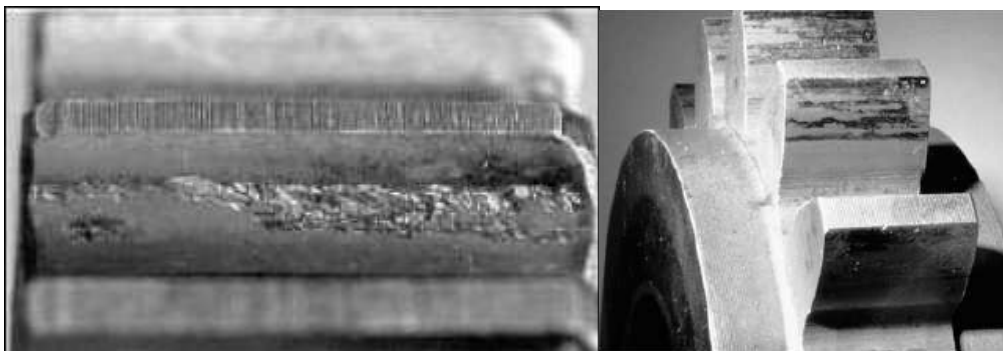
Fig. 4.2.7, 4.2.8 – Spalling e micropitting
