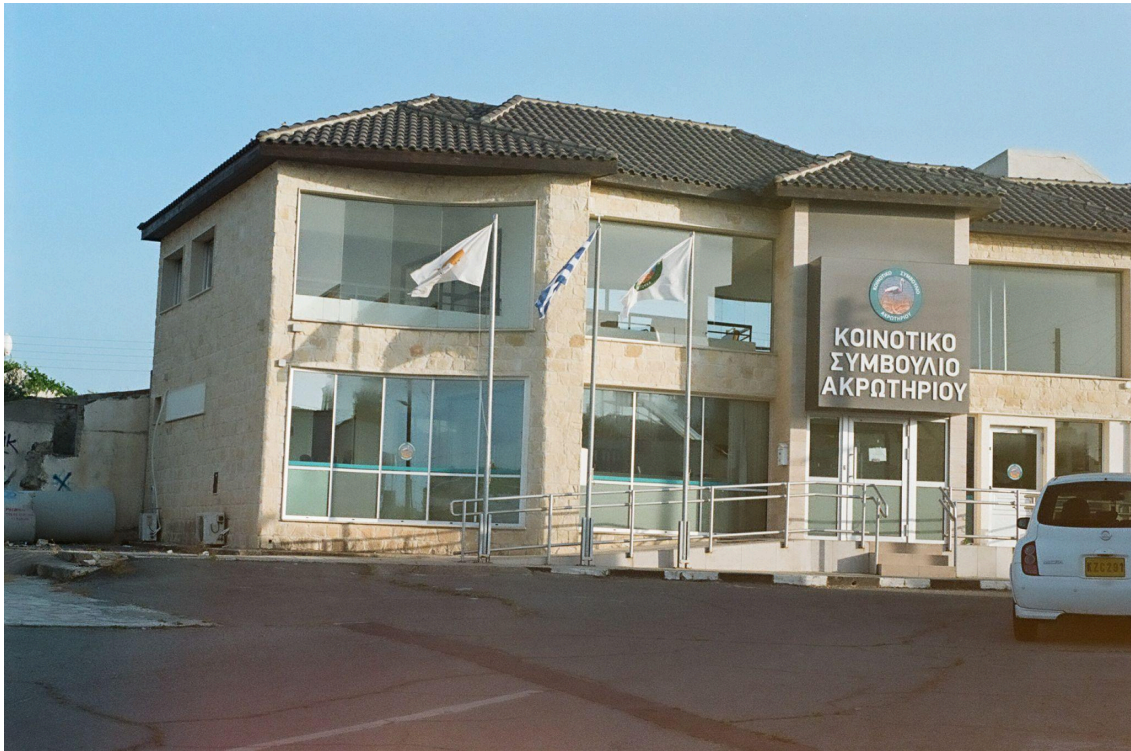
Image 7. Akrotiri Town Hall . Analog photograph [source: Ernesto Martellaro]
