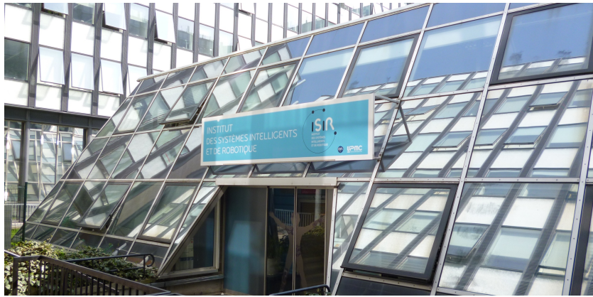
Figure 1: Photo of the ISIR pyramid in Jussieu, the main campus of the Faculty of Science of Sorbonne Université in Paris. Credit: (Université 2022)
