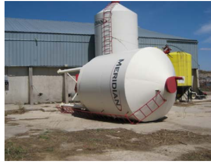
Fig. 1.1.6: Elevated tank overturning.
