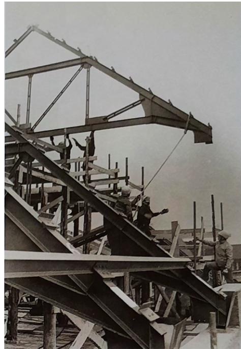
Figure 2.12: Truss placement
