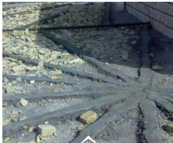
Figure 4.13 sloping with crushed brick
