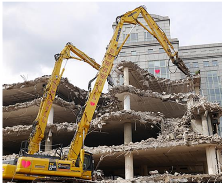
Figure 2.4 high reach arm demolition
