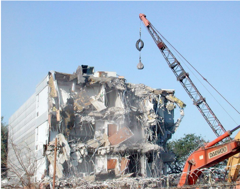
Figure 2.5 wreck and ball demolition
