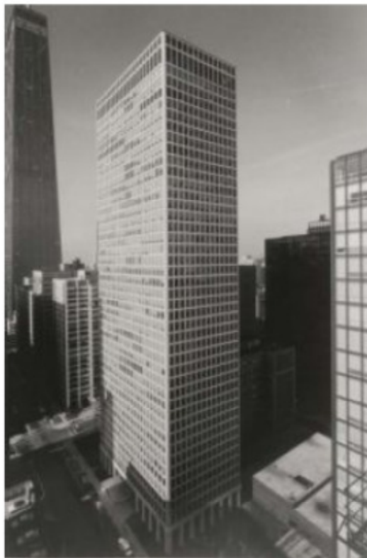
DeWitt-Chestnut Apartment building, Chicago, 1965, Khan
