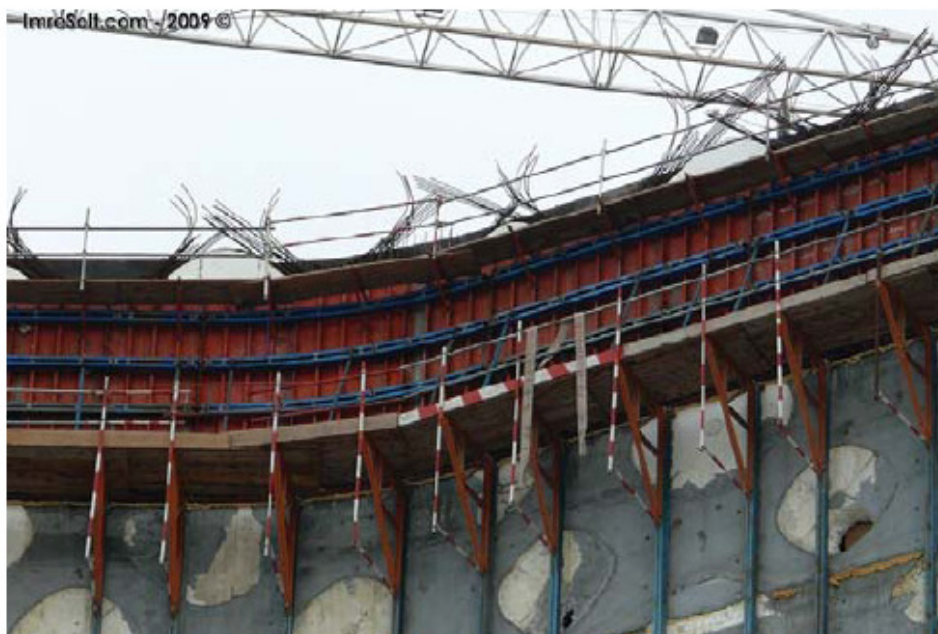
Step 2: casting a floor
