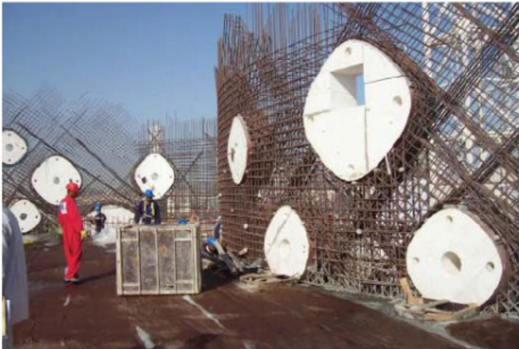
Step 1: polystyrene void forms in the rebar
