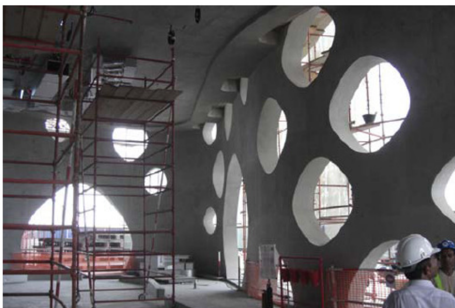
Interior under construction
