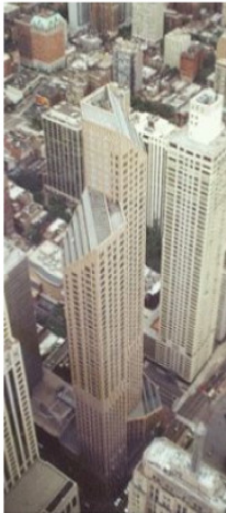
One Magnificent Mile building, Chicago
