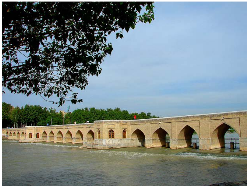
Figure 5-9: View of Juei Bridge
