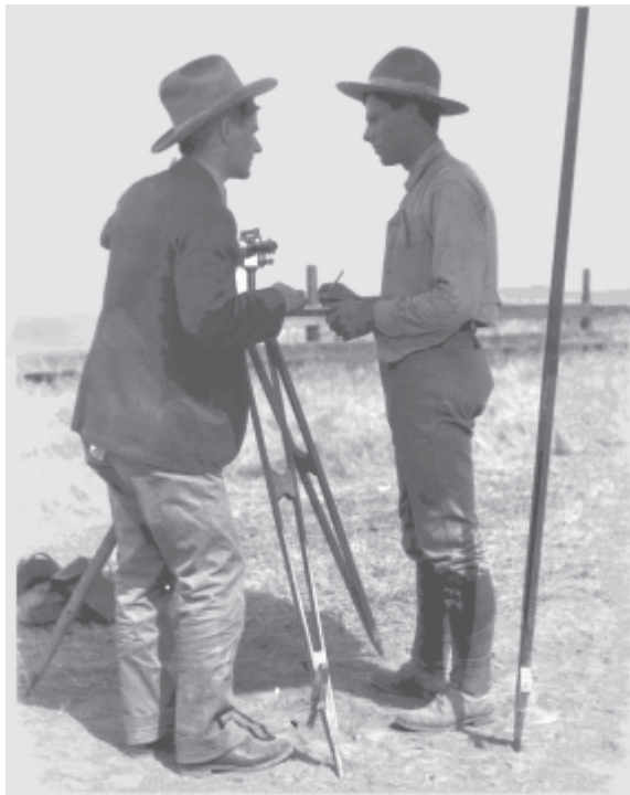
Figure 4-7: Spirit Levelling Survey in 1905 (Source: USGS website)
