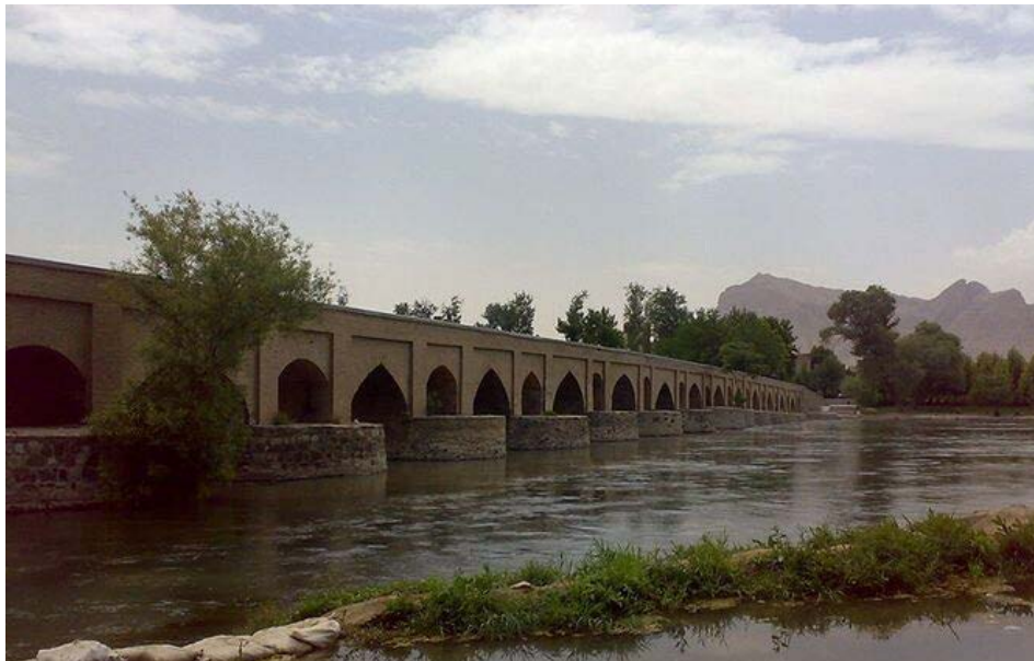
Figure 5-5: View of Marnan Bridge with the Existence of Water
