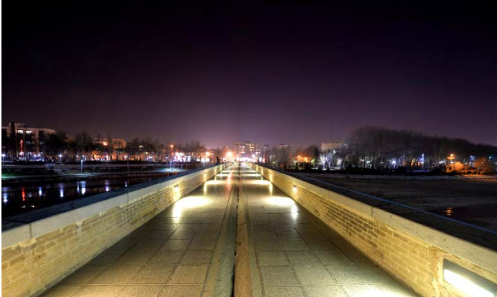
Figure 5-4: Marnan Bridge at Night
