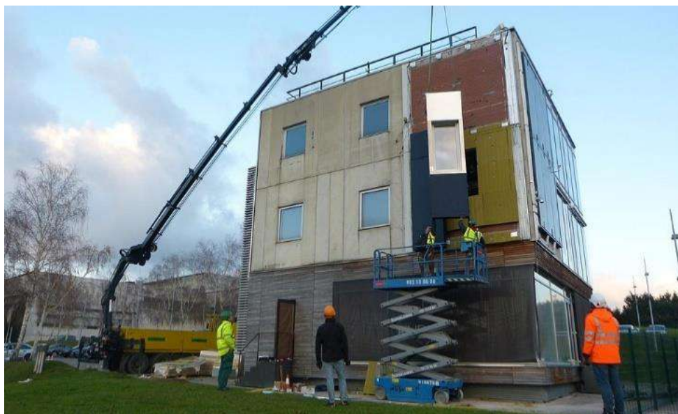
Fig. 1: Pre-validation of the RenoZEB modular façade in the KUBIK test Infrastructure (Bilbao, Spain) [Fonte: https://renozeb.eu/news/detail/article/pre-validation-of-the-renozeb-modular-facade-in-the-kubik-test-infrastructure-bilbao-spain.html ]
