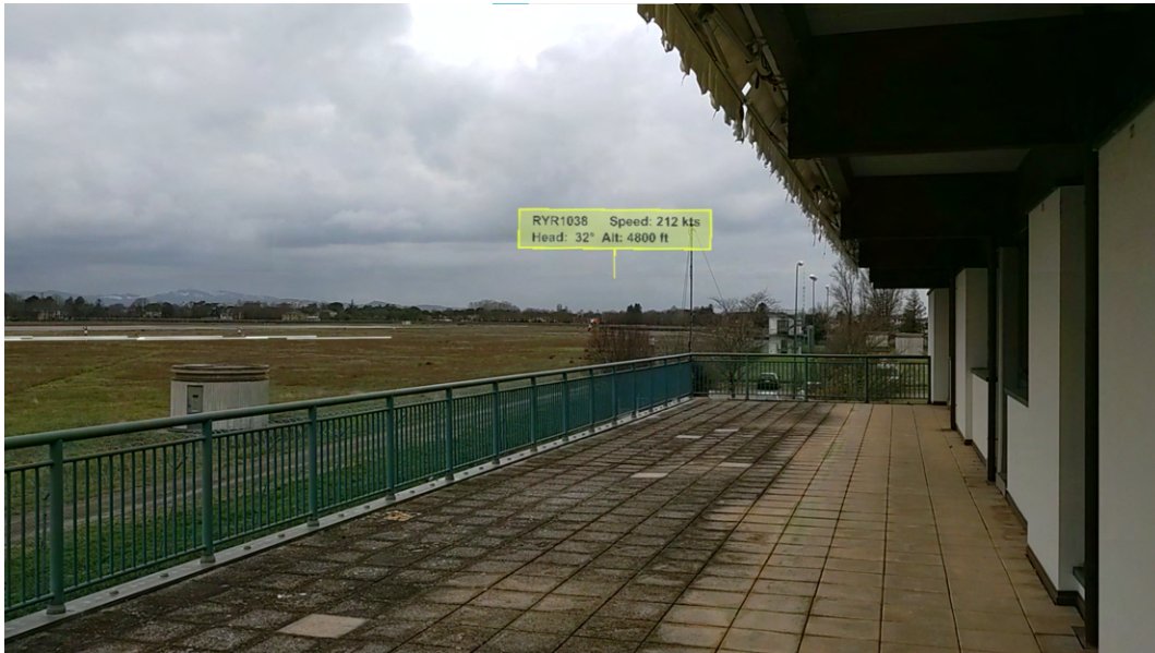
Figure 6.3: Terrace visibility over the runway.
