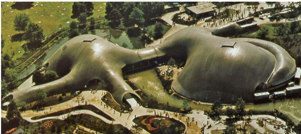
Figure 3.6 - Mannheim Multihalle timber gridshell by Otto Frei during construction (top-left) and digital model (top-right) (Liddell, 2015)
