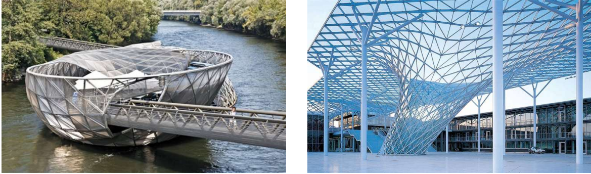
Figure 3.8 - Examples of freeform gridshells: the Murinsel Gridshell and the roof of the Fiera di Milano
