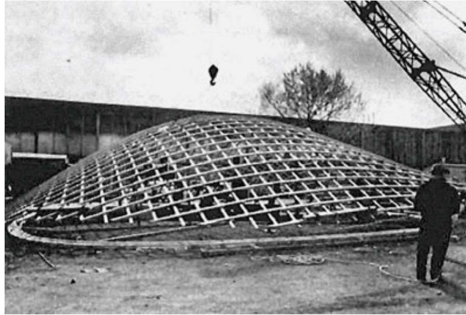
Figure 3.5 - Frei Otto's first timber gridshell in Essen, Germany, 1962 (Leung)
