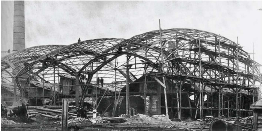
Figure 3.2 - Vladimir Shukov's metal plate-rolling production hall, Vyksa, Russia, during construction, 1897 (Leung)
