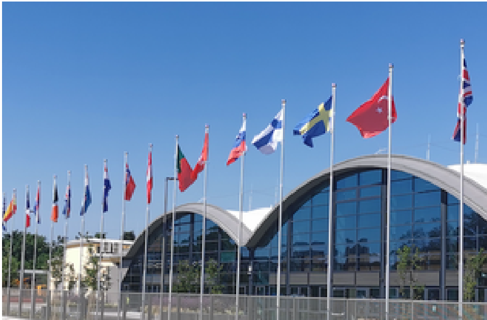
Figure 5.2: LEONARDO is to be hosted in Bologna, on the redeveloped site of the former Manifattura Tabacchi (tobacco factory) [73].
