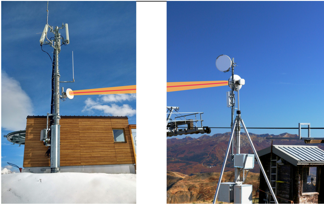
Figure 3.2: CML antennas over the Appennine crest, over M. Cimone (left) and Corno alle Scale (right), the two highest peaks of Emilia-Romagna. In yellow, an artistic impression of the electromagnetic beam around the line connecting the two antenna dishes (red line).
