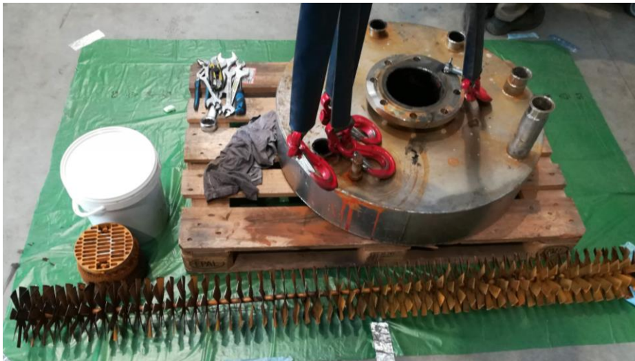
Figure 4.6: The dismantling process of scrubber with the insertion of new impeller.
