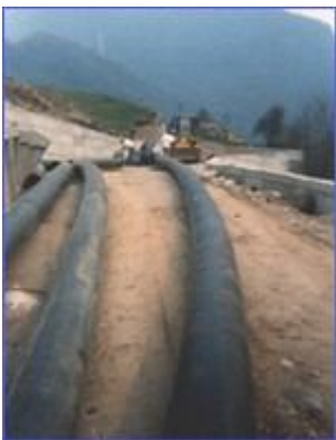
Fig.5 Tubi in PEAD posati in opera.
