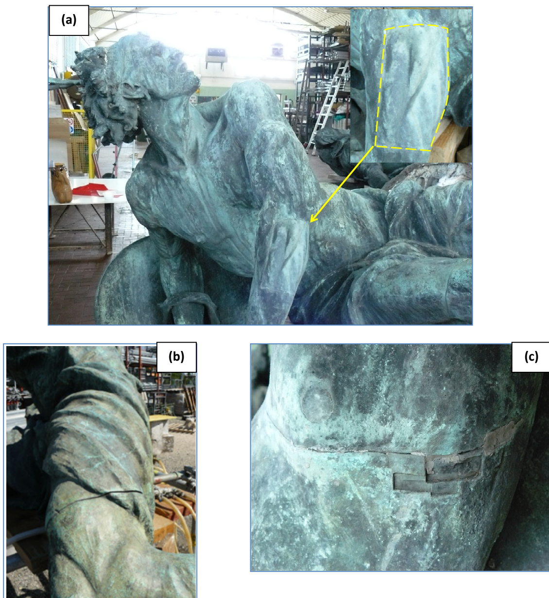
Fig. 1.11 - Metal patch for fixing the damage due to bombing during World War II (a) and assembly between different sections in Omo statue (b, c)
