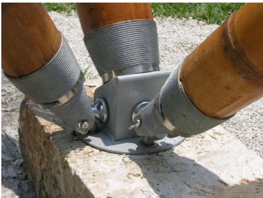
Figura 78 Bamboo Pavillon, Keystone Footers, Guaduatech Project.
