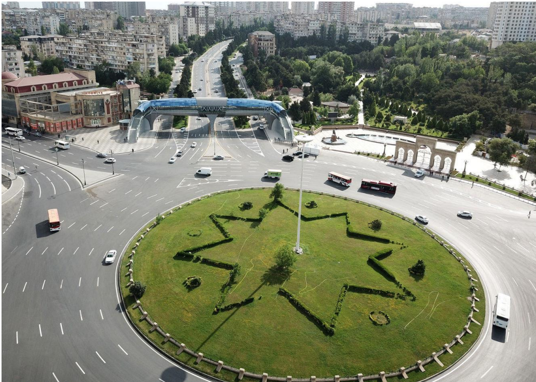
Figure 17. Special part of the “Ukraine” roundabout.
