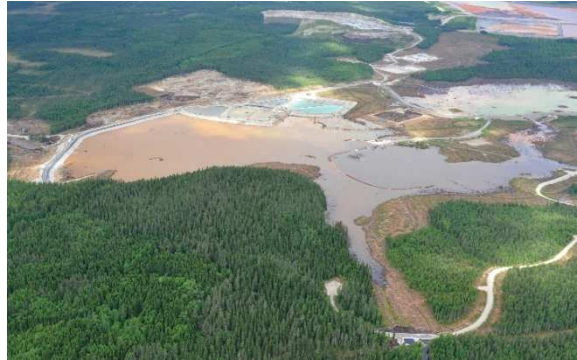
Figure 5. Mine tailings dam failure , Brazil (mining-technology.com)
