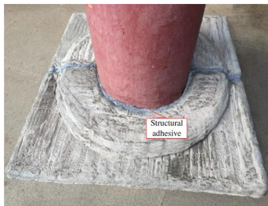
Figure 49: Installation of the Plinth 2
