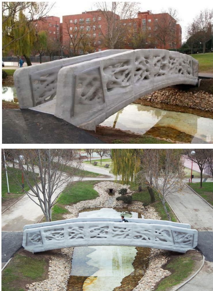
Figure 28: Castilla La Mancha 3D Printed Pedestrian Bridge
