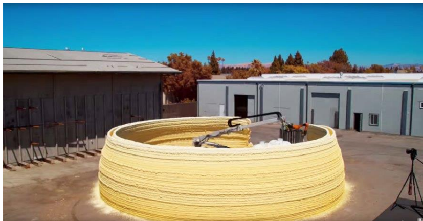
Figure 35: The Dome Constructed by DCP
