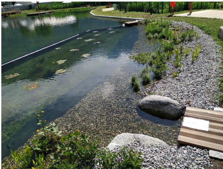
Figure 32: Skimmer tools for pre-filtering - Pinzolo Biolake
