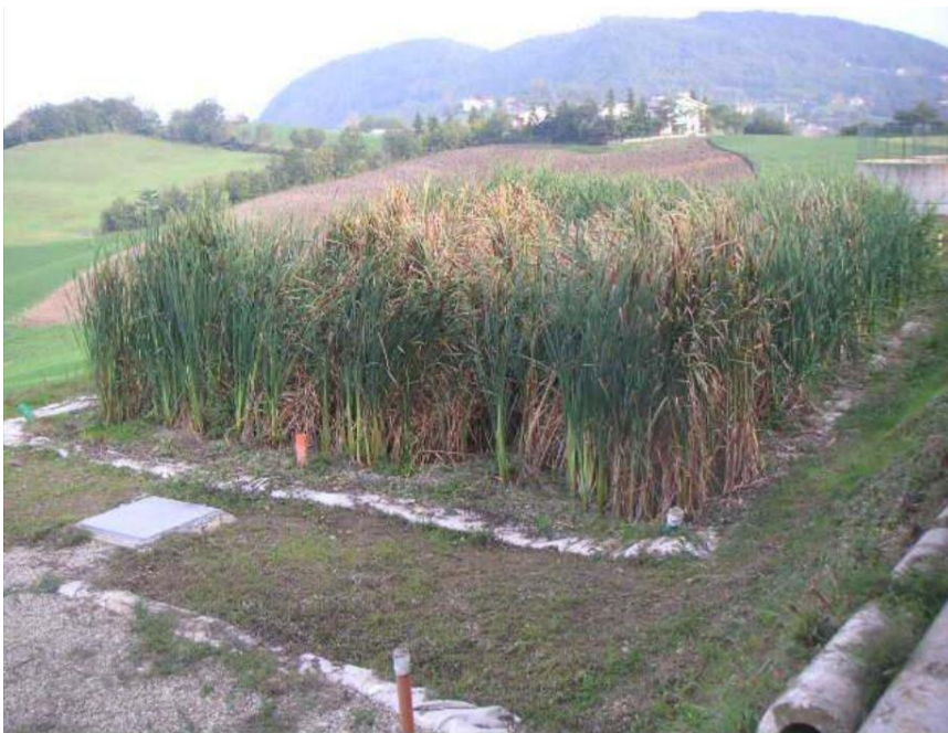
Figure 10: constructed wetland for treatment of dairy's wastewaters (Salto di Moltese MO) (Lajo, s.d.)
