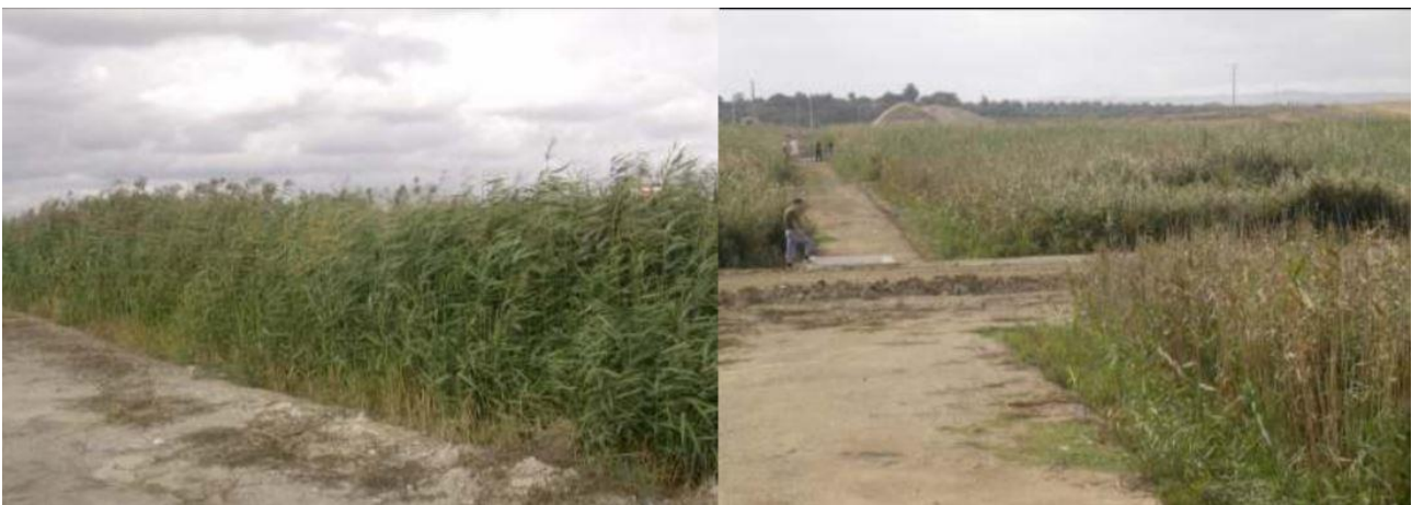
Figure 8: Constructed Wetland for treatment of small community municipal wastewater (32000 PE, 3 ha) (Lajo, s.d.)
