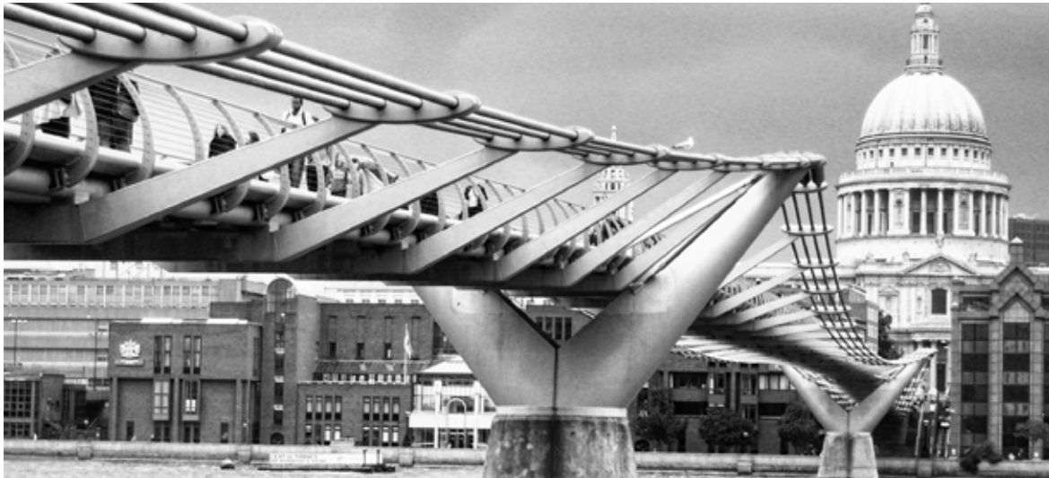
F5: httpwww.chsrentals.comwp-content/uploads/201509/millennium-bridge-london.jpgw=240 Vista globale S-E
