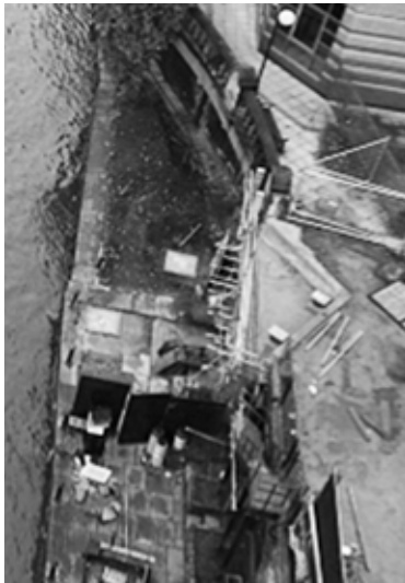
F11: http://www.suaveairphotos.co.uk/general/2/EricWrightIrwelFootbridge/Fondazioni Nord
