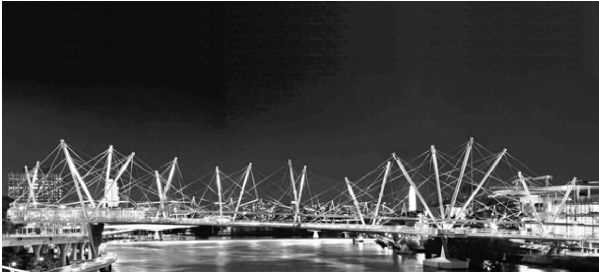
F5: http://c1038.r38.cf3.rackcdn.com/group1/building5510/media/Kurilpa_12_ChristopherFrederickJones1.jpg Vista laterale N-O
