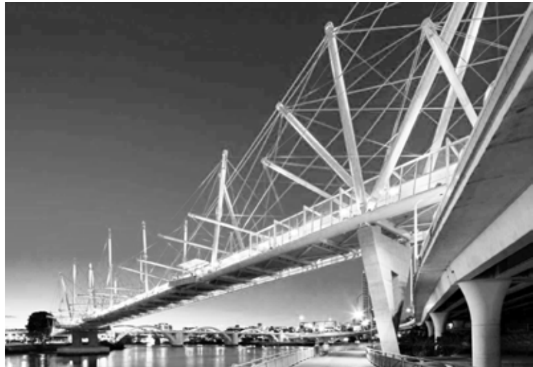
F11: http://1.bp.blogspot.com/-ZTAkNP138MI/UU2GzcKcHsl/AAAAAAAAcLU/b7sWHIhbqaA/s1600/Kurilpa+Bridge+by+Cox+Architecture04.jpg Vista globale intradosso
