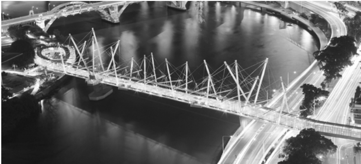
F9: http://c1038.r38.cf3.rackcdn.com/group1/building5510/media/Kurilpa_12_ChristopherFrederickJones1.jpg Vista globale Est
