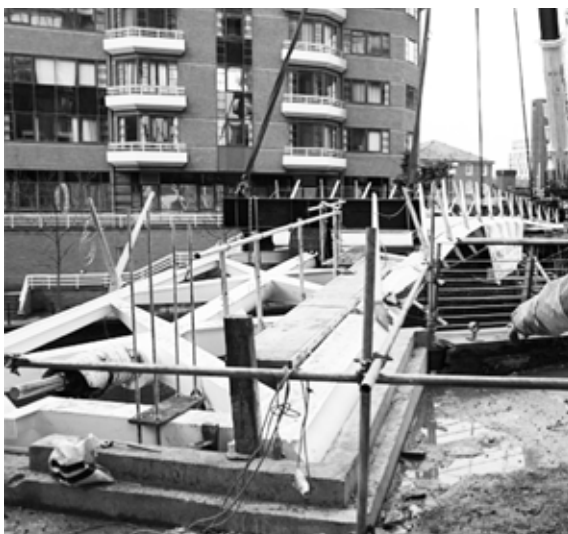
F8: http://www.suaveairphotos.co.uk/general/2/EricWrightIrwelFootbridge/ Montaggio spalla Sud
