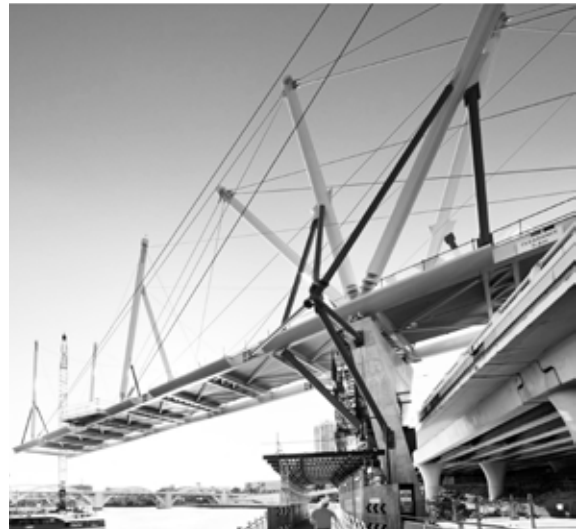
F13: http://www.coxarchitecture.com.au/wp-content/uploads/2009/01/406081_00_N205_medium.jpg Vista Est appoggio INTERNO N-E con supporti provvisori
