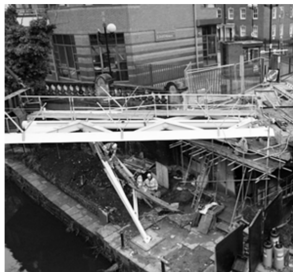
F9: http://www.suaveairphotos.co.uk/general/2/EricWrightIrwelFootbridge/ Montaggio spalla Nord
