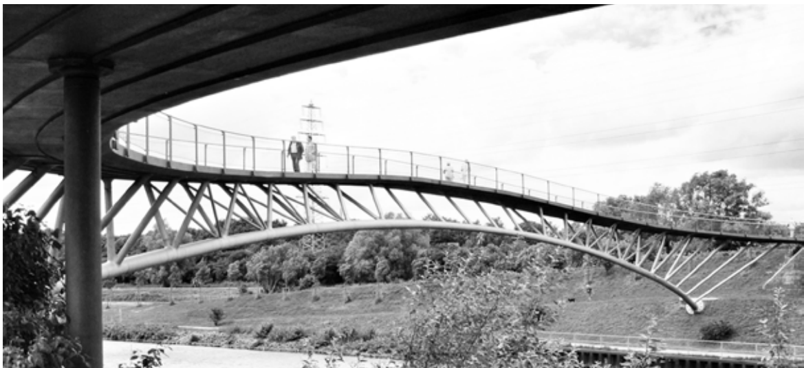
F6: https://hiveminer.com/Tags/hausripshorst Vista laterale S-E
