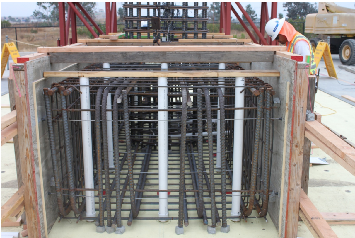
Figure 2.4: Footing during construction
