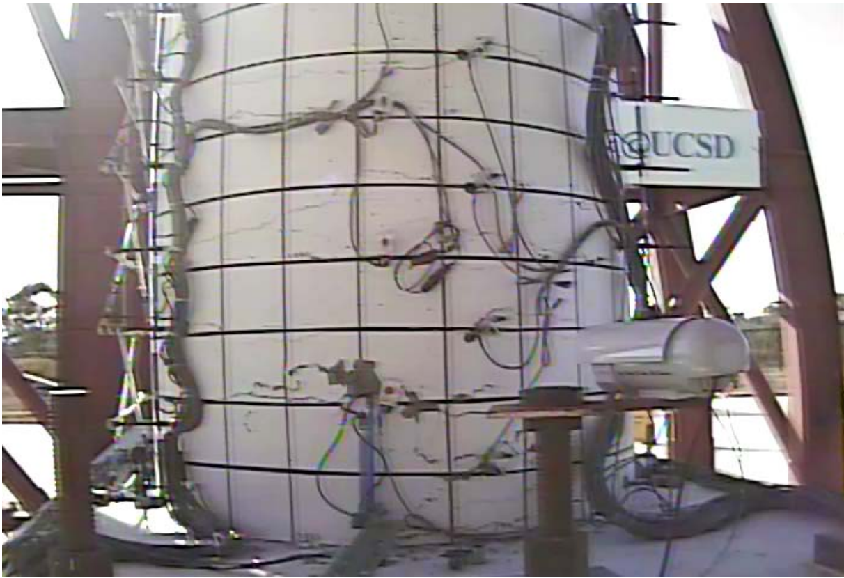
Figure 4.27: Column base post-EQ3
