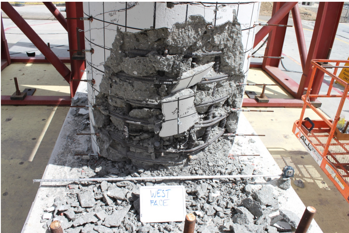
Figure 6.2: West face of the column base at the end of testing
