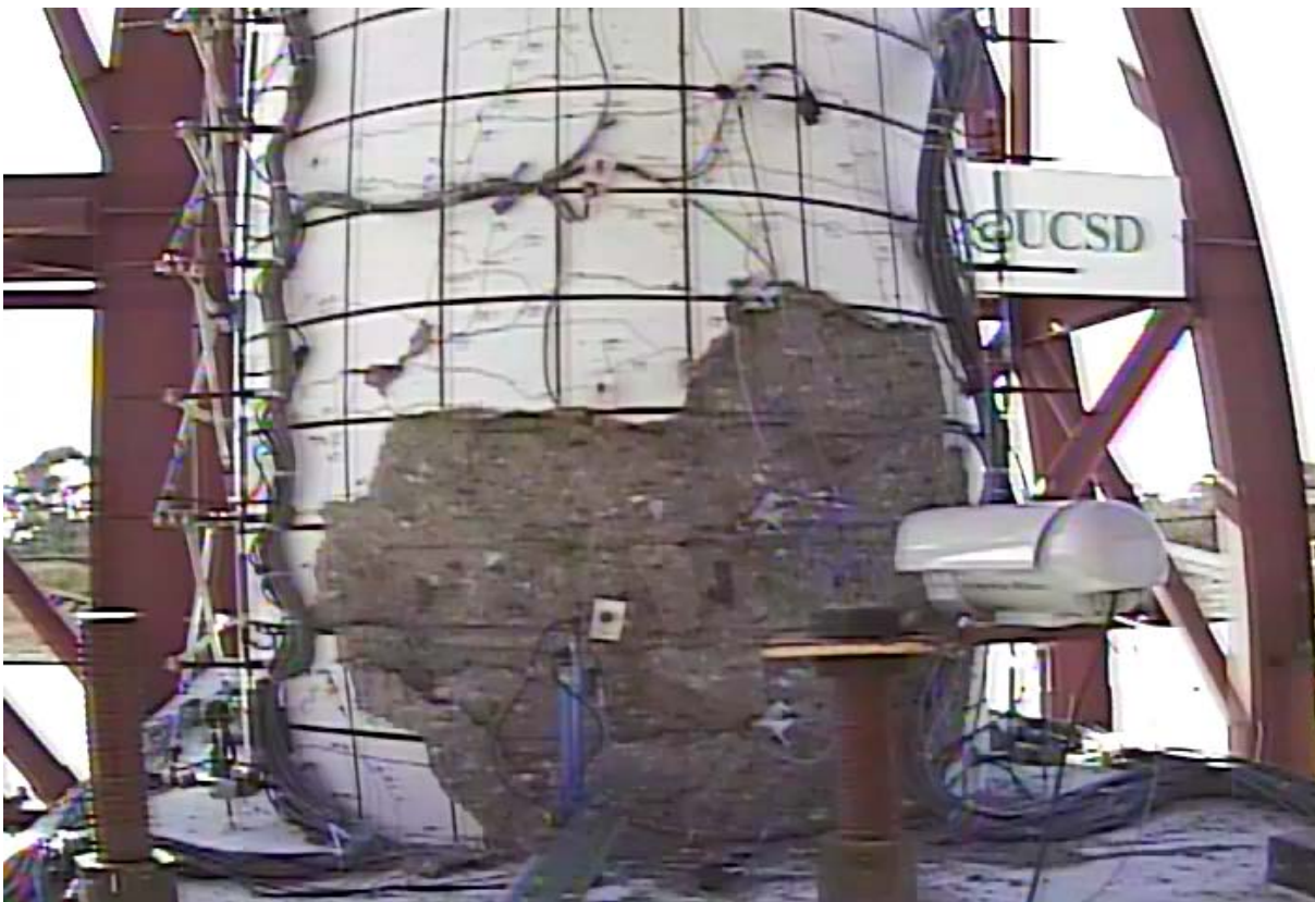
Figure 4.63: Column base post-EQ6
