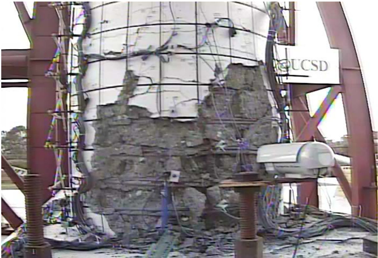
Figure 4.87: Column base post-EQ8
