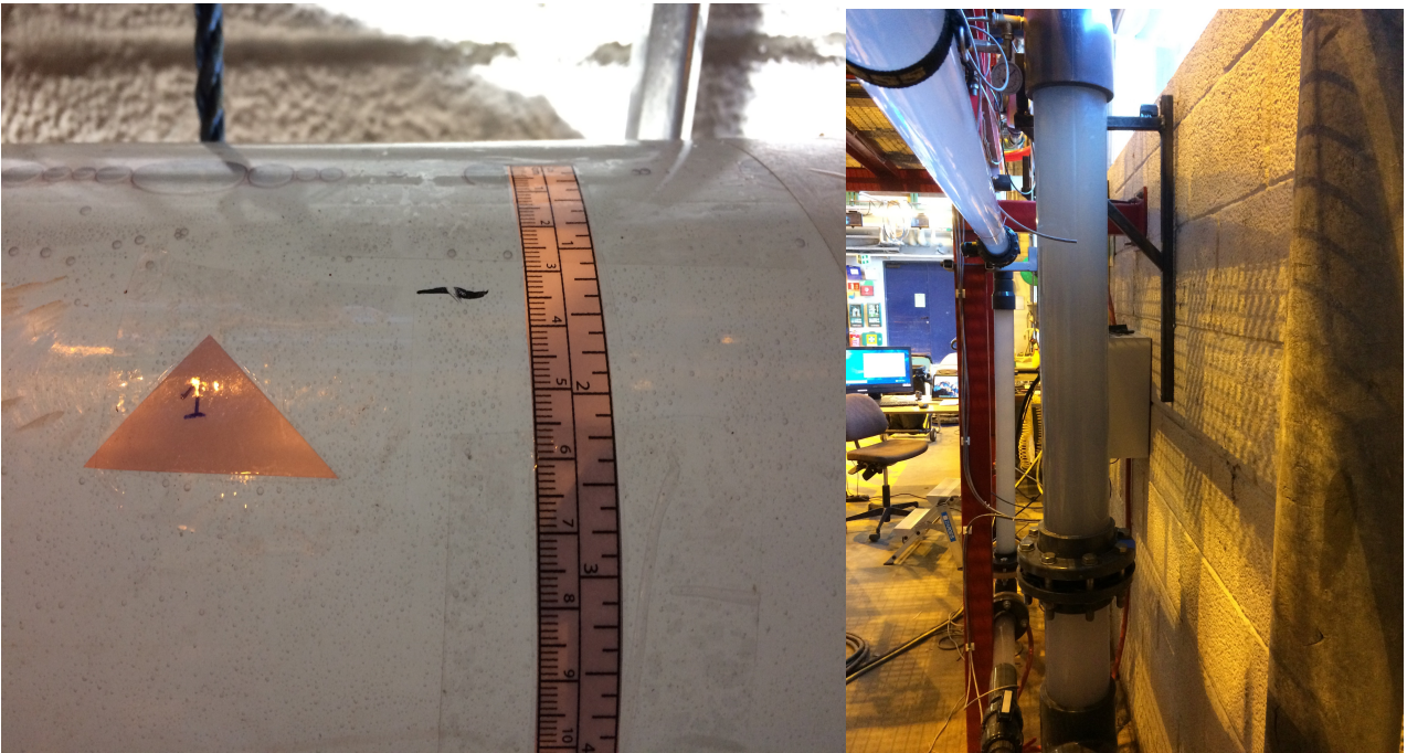
Figure 6.12: Pipes after 700 seconds injecting 20,77 \text{ m}^3/\text{h} when water displacing oil
