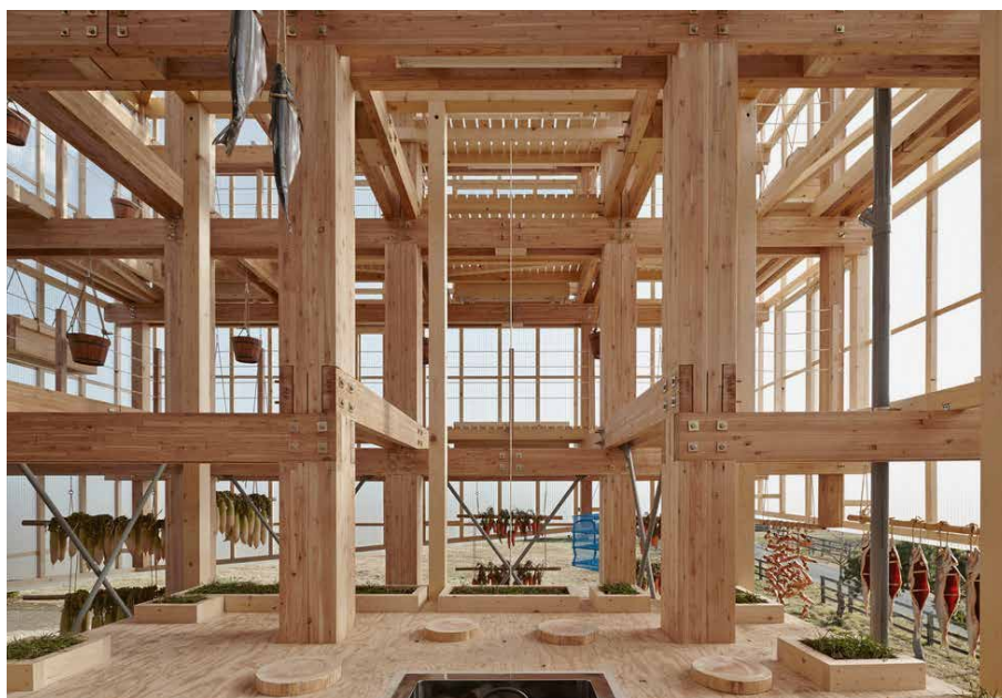
Foto di Nest we grow, Hokkaido, studio Kengo Kuma + College of environmental design U.C. Berkeley. Legno lamellare
