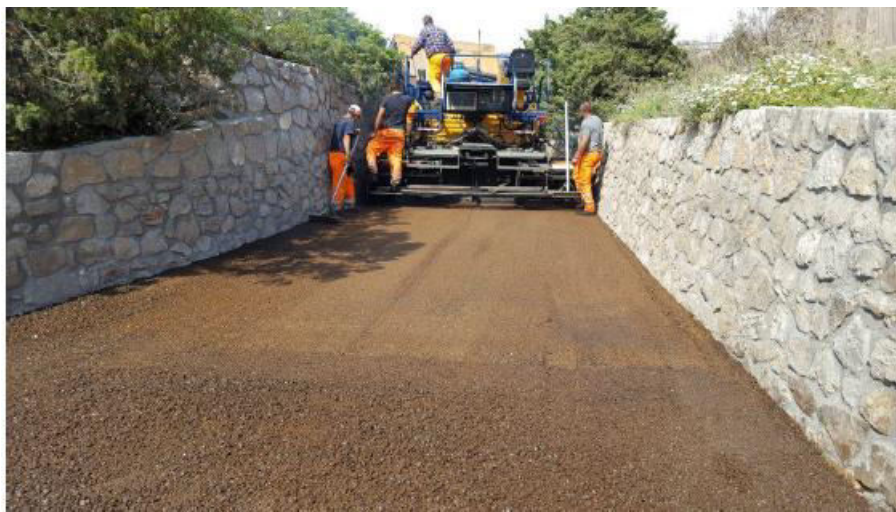
Figure 1-19 Laying of transparent bituminous conglomerates
