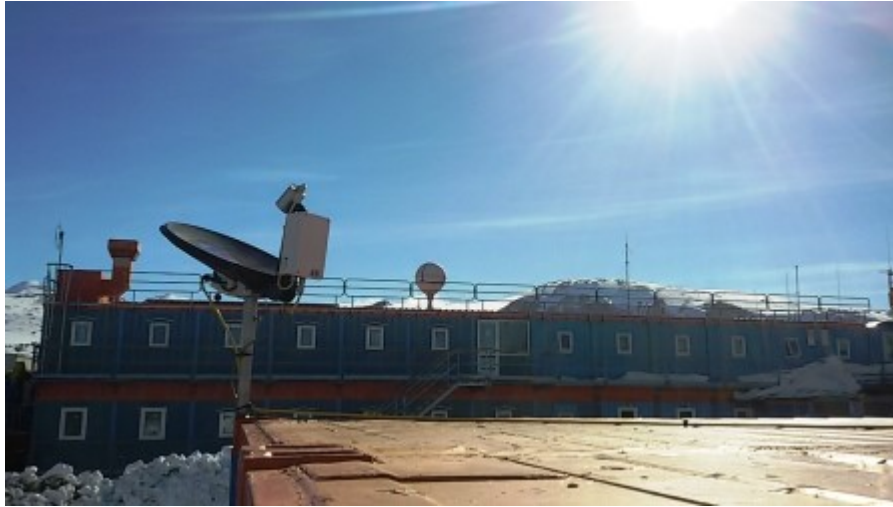
Fig. 3.3: Micro Rain Radar at Mario Zucchelli research station on the roof of the logistic container.
