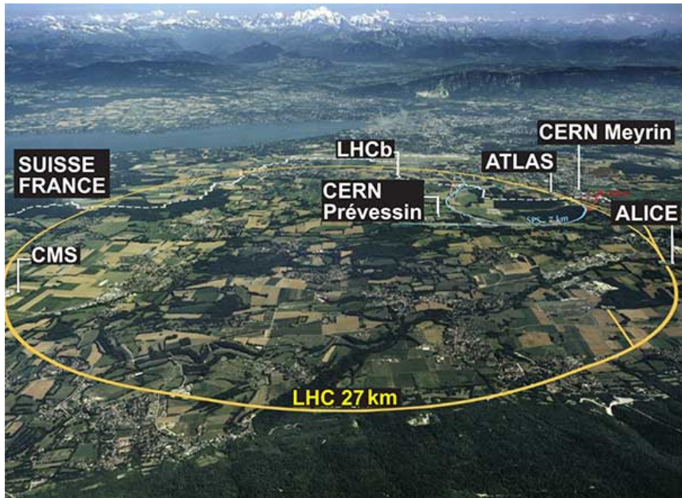
Figure 2.1: LHC ring. Aerial view.
