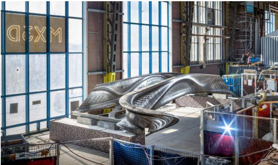
Figure 1. 3D printed steel bridge the at MX3D [1]
