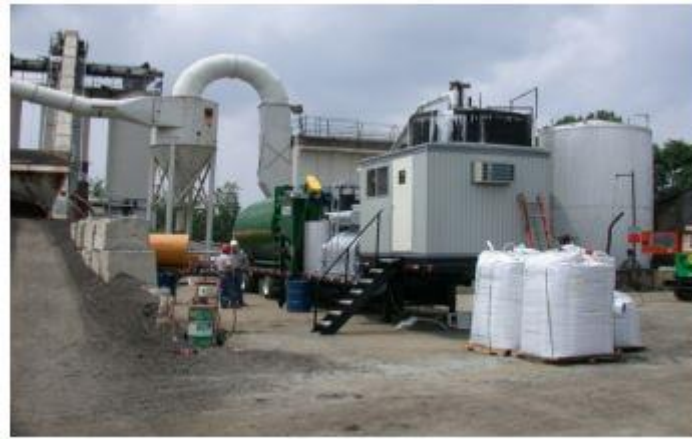
Figure 2.13 -Wet Process On-site.
