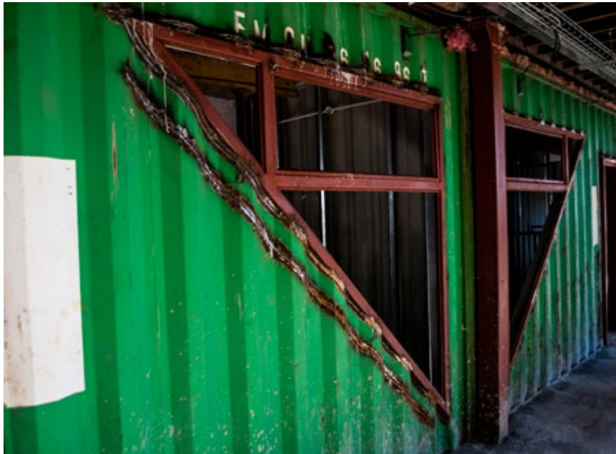
FIGURE 1.9 - Cut and reinforcements for window opening - Drivelines Studios
