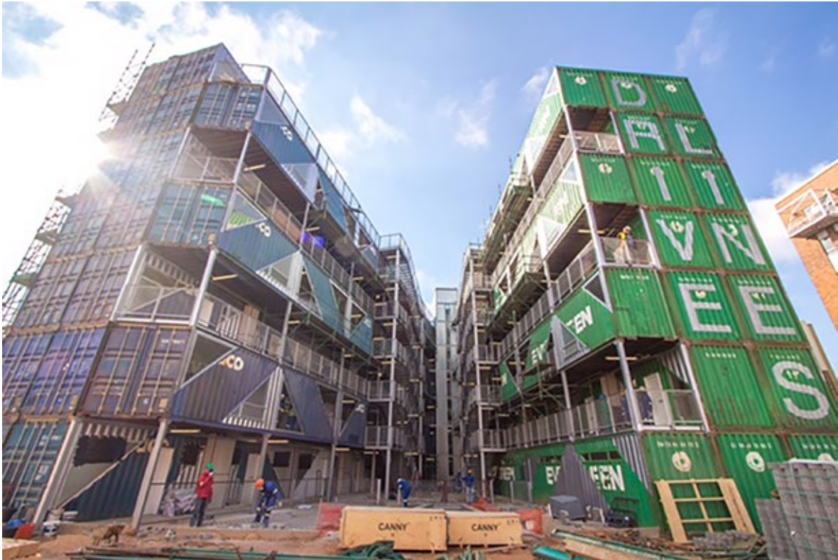
FIGURE 1.16- Drivelines Studios - Courtyard view - source LOT-EK studio
