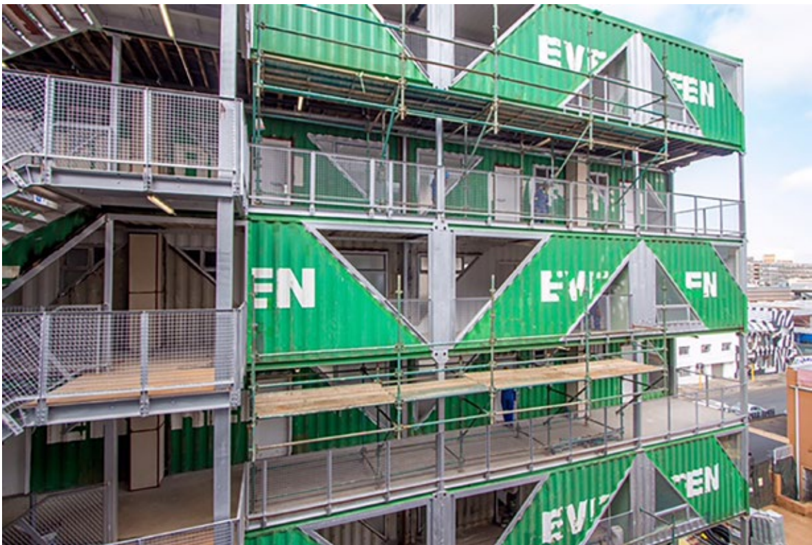
FIGURE 1.17 - Drivelines Studios - Walkway view - source LOT-EK studio
