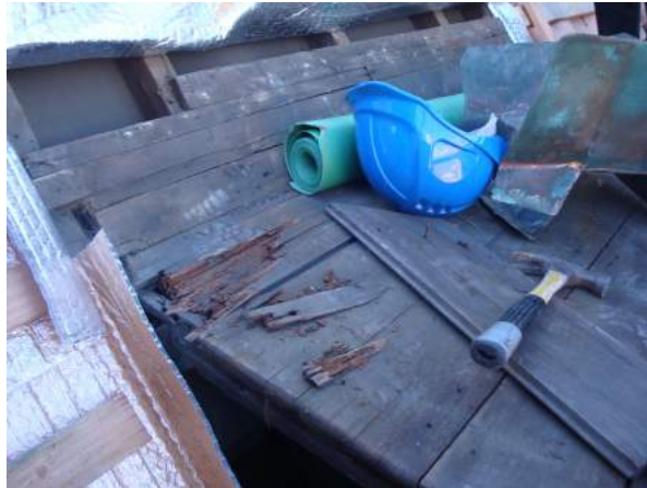
Figures 4.25. Removal of the damaged battens
