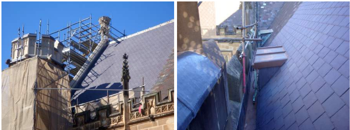
Figures 4.26, 4.27. Installation of a new roofing system
