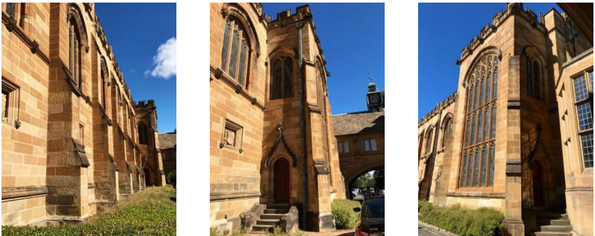
Figures 4.7, 4.8, 4.9. Buttresses and projecting bay on the right side wall
