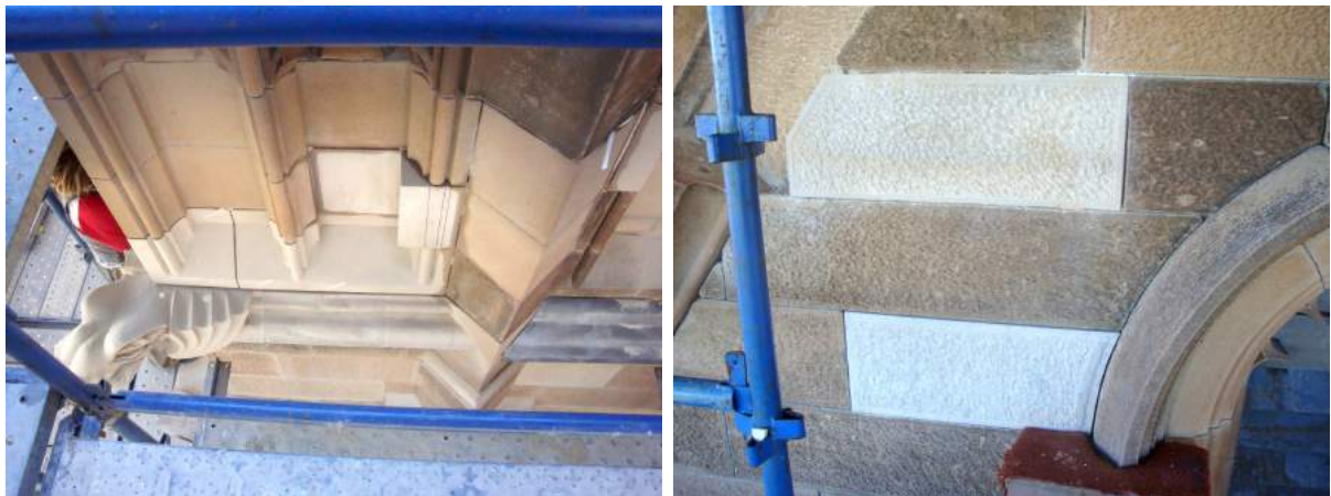
Figures 4.19, 4.20. Replacement of the damaged stones
