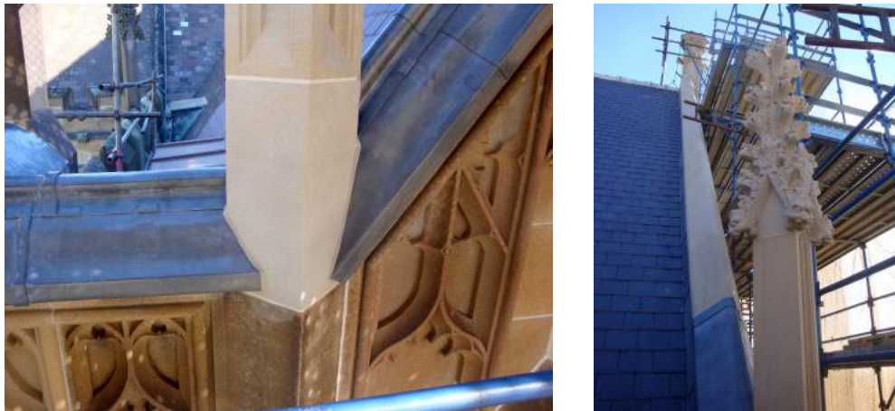
Figures 4.23, 4.24. Replacement of the damaged and unstable pinnacles
