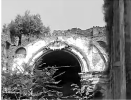
Vista interna, abside
