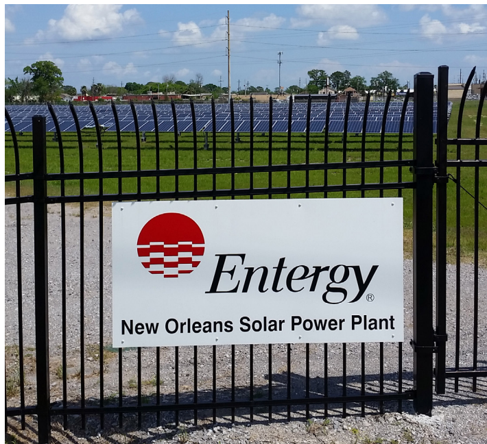
Fig. 4.1: Entergy Solar Farm in New Orleans (courtesy of Entergy Inc.)
