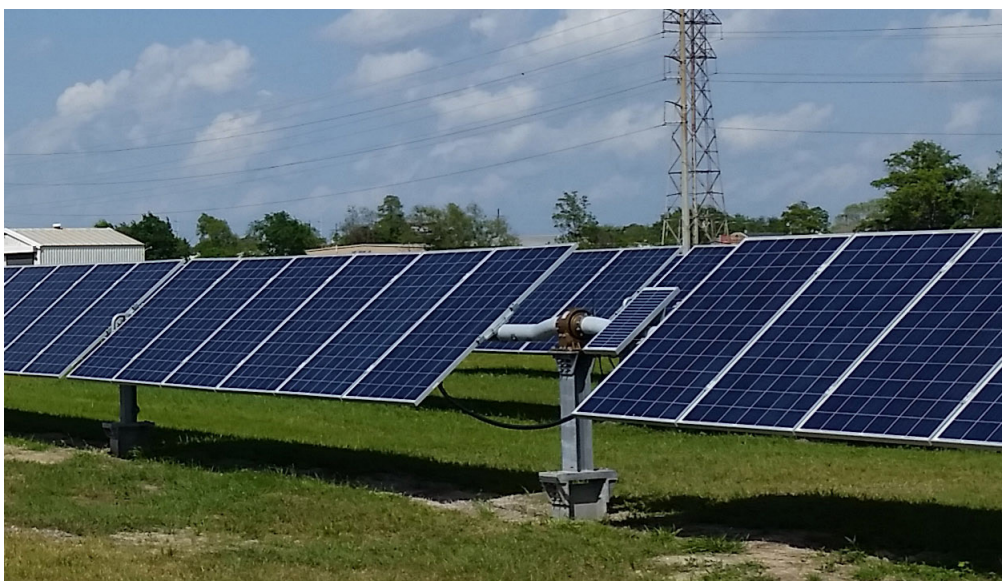
Fig. 4.2: A detail of the PV panel dedicated to the tilt of the whole row of panels (courtesy of Entergy Inc.)
