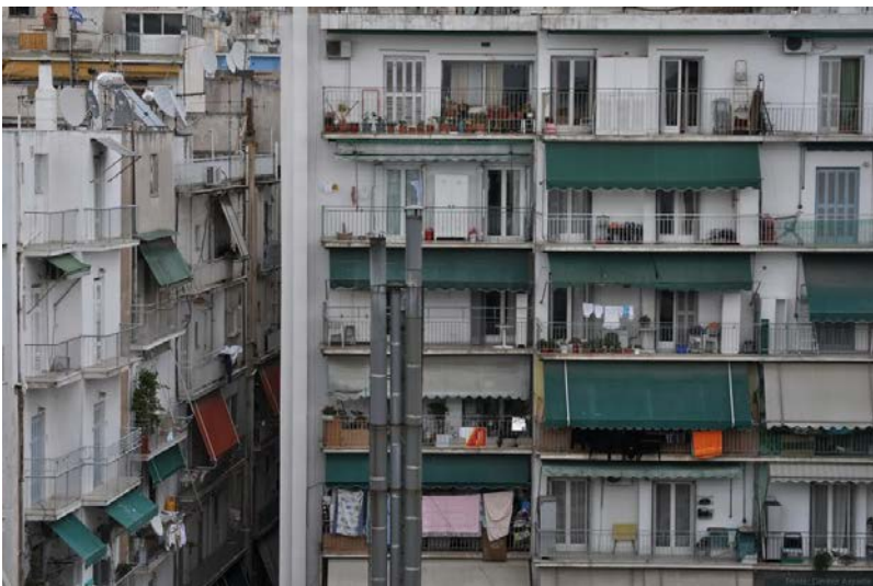
Figure 2.1 Building in the district of Kypseli, Athens (source: google images)
