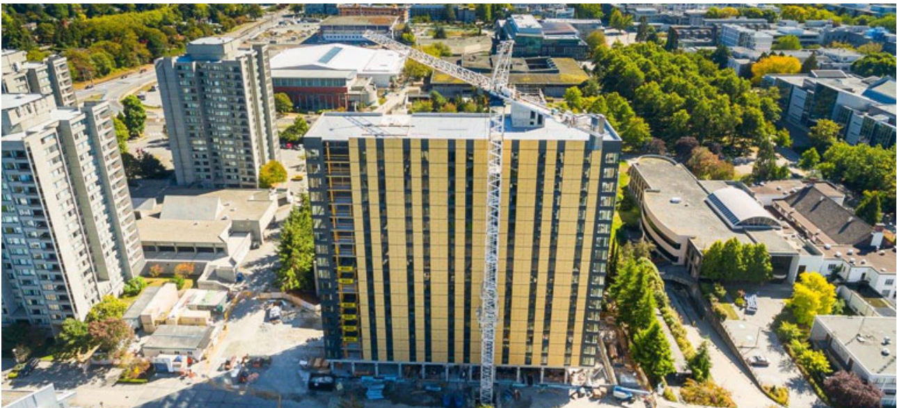
Figure 7.15 UBC's tall wood building, Brock Commons (source: www.news.ubc.ca )
