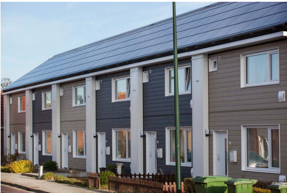
Figure 2.5 Oud-Vossemeer, example of Energiesprong's work (source: www.energiesprong.nl )
