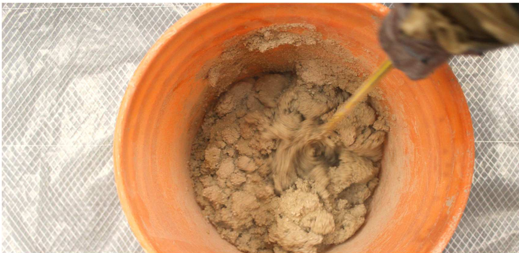
Fig. 26. Preparation of a mixture of plaster.
